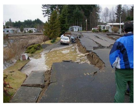
Figure 4: Seismic Induced Ground Failure in Mw 9 Earthquake, Japan, 2011
