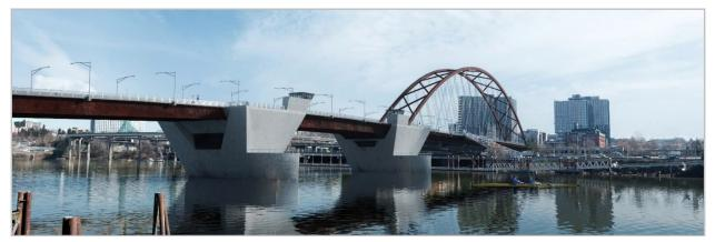
Figure 6. Preferred Alternative with Bascule Movable Span (Cable Stayed East Approach)
