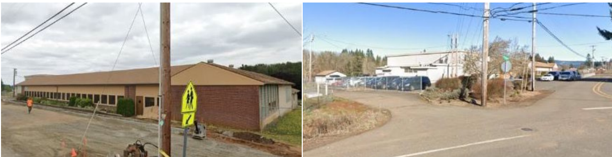
Figure 9. School Buildings on Proctor Road
