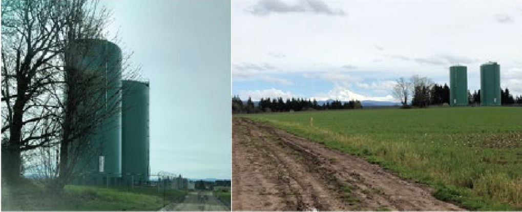
Figure 10. Pleasant Home Water District Towers
