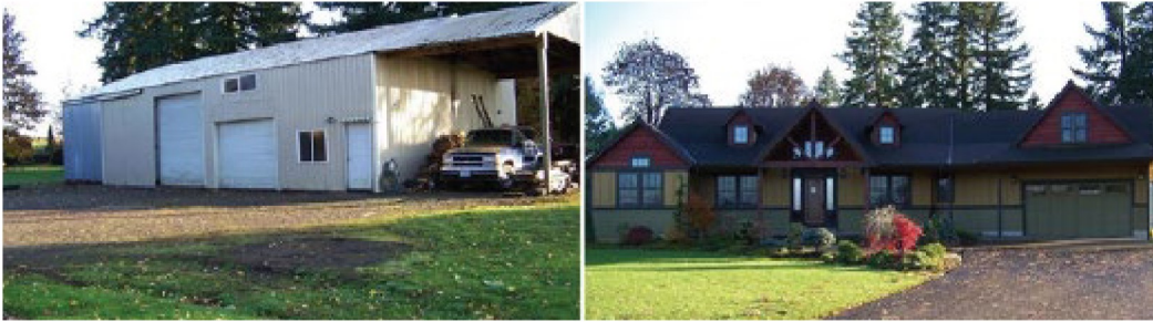
Figure 3. Residence and Accessory Structure on Bluff Road
