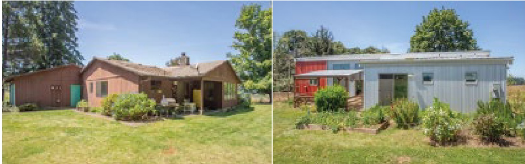
Figure 4. Residence and Accessory Structure on Proctor Road
