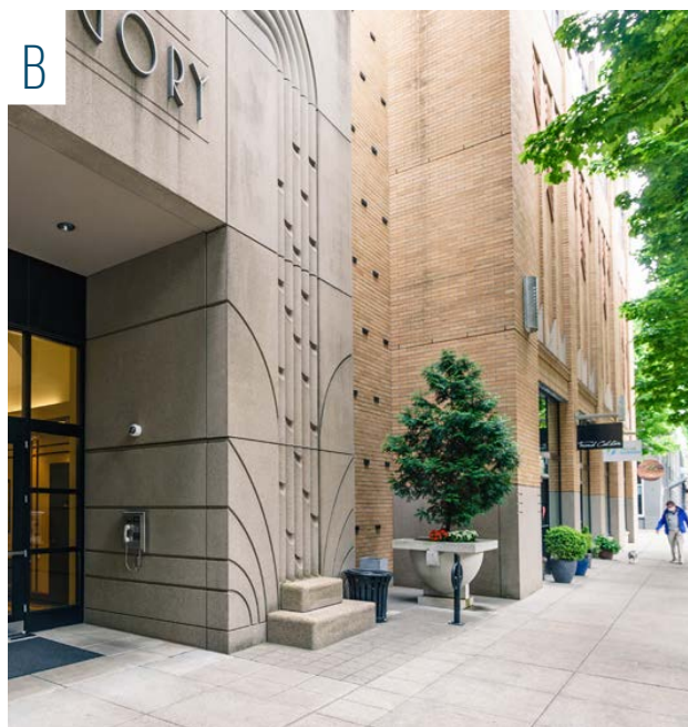
Integrating detail and craftsmanship at the ground floor. This multistory building utilizes durable materials at the base, increasing levels of texture and interest around the lobby entrance. Pearl , NW 11th and NW Glisan
