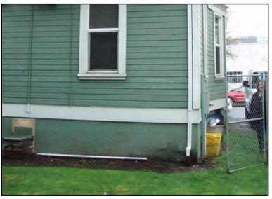
1.04 The concrete basement walls at 732 NE Couch exhibit the same poor concrete quality and moisture intrusion issues as 722.
