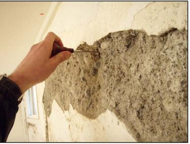
1.03 On the other side of this wall, a gutter downspout routes water to a drain line running along the exterior side of this wall.
