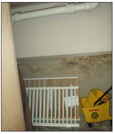
1.05 This wall could be picked apart by hand, revealing visibly moist concrete behind the surface.
