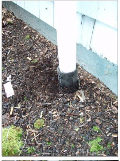
1.07 This downspout at the southwest corner of 722 leads to a drain line featuring a typical bell as well as a clean out. This drain line appears blocked/ clogged, as standing water was visible at the surface of the bell.
