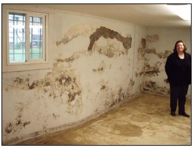
1.02 The turn-of-the-century concrete could easily be picked apart by hand. This is typical for basement walls of this vintage.
