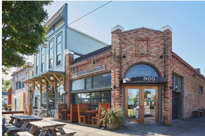
Historic resources in the Woodlawn Conservation District.
