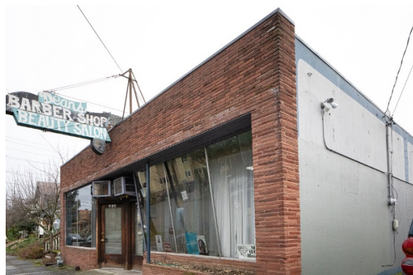
Dean's Barber Shop and Beauty Salon is Portland's oldest continuously operating Black-owned business. While the City sponsored a National Register nomination for the building in 2021, there are few tools available to protect institutions from displacement. Photo by Intisar Abioto.
