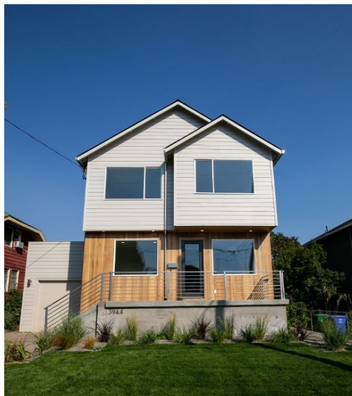
This “1922 bungalow” was altered in 2018 without meeting the threshold necessary to require a demolition permit. A new definition of demolition specific to historic resources is recommended.
