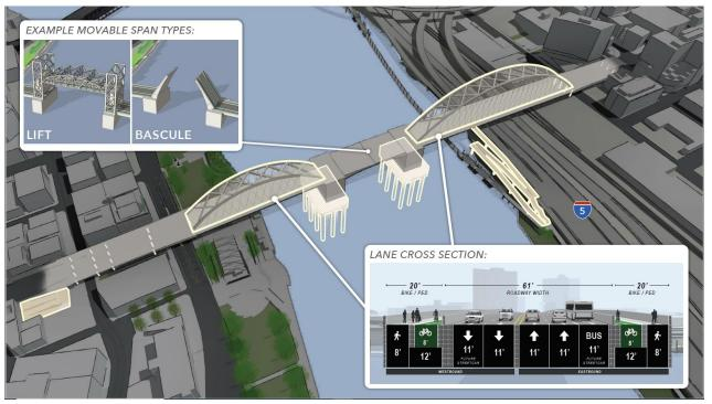
Note: The Draft EIS Long-span Alternative included multiple bridge types for both the east and west approach. This figure shows only the tied arch option.
