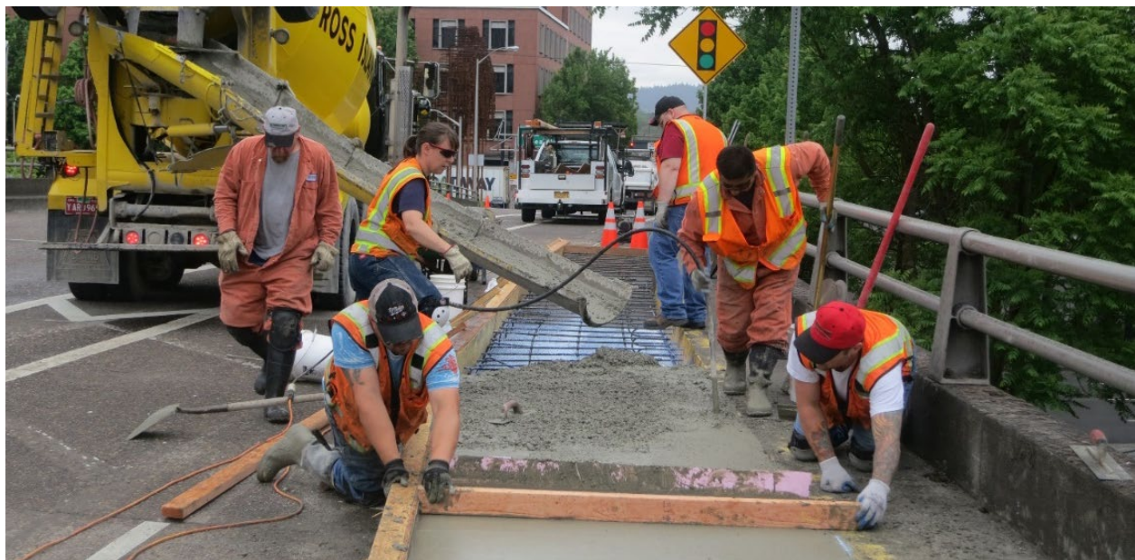
Figure 3: Picture of crews constructing a sidewalk on Hawthorne Bridge
