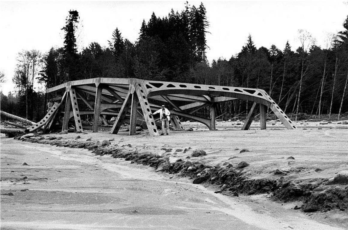
Figure 85 - The Saint Helens Bridge on Highway 504 in Washington was carried over a quarter mile downstream by a lahar from the 1980 Mount St. Helens eruption. Photo by R.L. Schuster for the United States Geological Survey.
