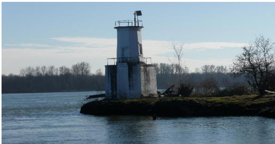
Figure 156 - The Warrior Rock Lighthouse guides ships on the Columbia River from an eastern point on Sauvie Island. It is the smallest lighthouse in Oregon. Photo from the Sauvie Island Community Association .
