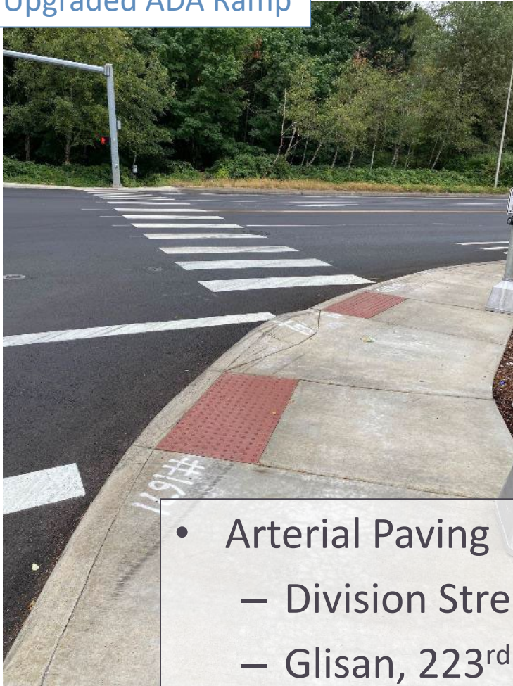
Upgraded ADA Ramp
