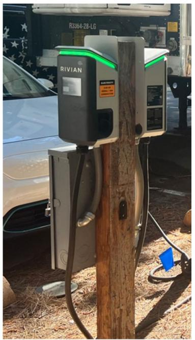
Figure 1. Above is an example of the proposed Electric Vehicle (EV) charging stations for Rooster Rock State Park. The above is from Yosemite National Park
