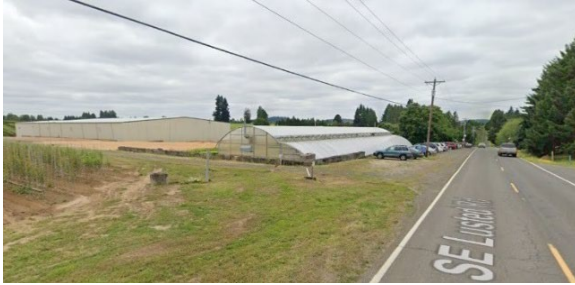
Figure 14. Surface Nursery Headquarters
