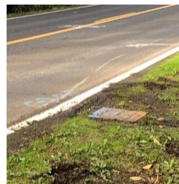
Figure 3. Existing Drain in Lusted Road ROW
