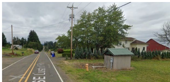
Figure 19. Roadside Pump Station and Utilities
