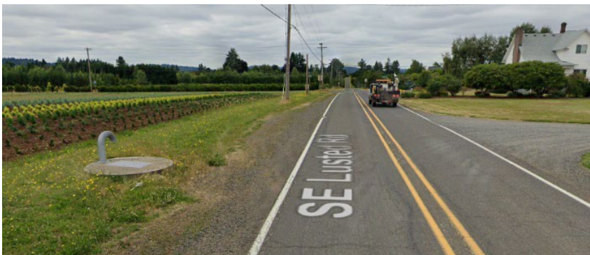
Figure 2. Example of Existing Air Vent and Access Vault (left) within Lusted Road ROW
