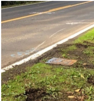
Figure 13. Existing Drain in Lusted Road ROW
