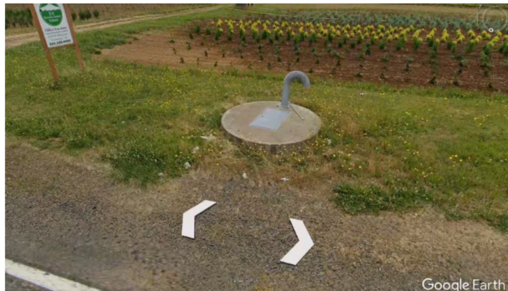
Figure 18. Existing Roadside Vent
