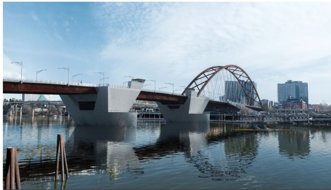
Pictures show conceptual renderings of the Preferred Alternative, the Replacement Long Span. The images show two examples of what a long span bridge could look like (cable-stayed pictured at the top and tied-arch picture at the bottom).
