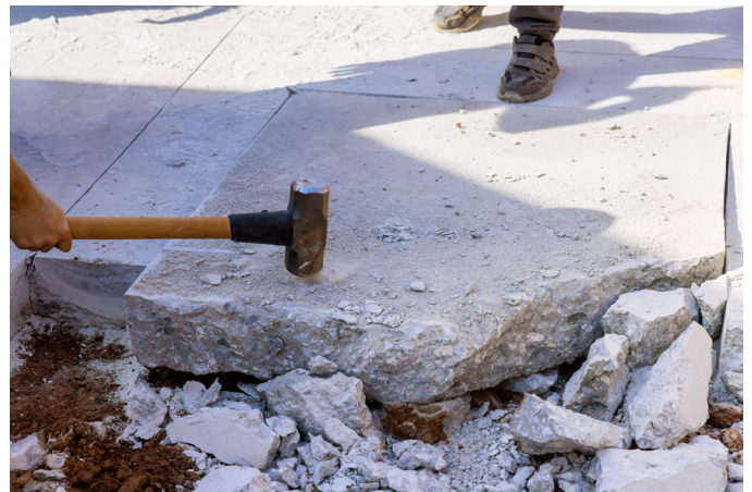
Image description: Concrete is broken apart by people using large hammers.
