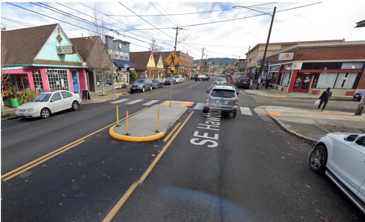
Figure 25: Example Pedestrian Crossing with a Refuge Island and Curb Extensions (Portland, Oregon)
