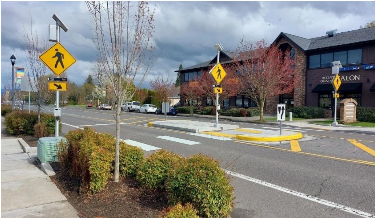
Figure 24: Typical Enhanced Pedestrian Crossing with a Refuge Island
