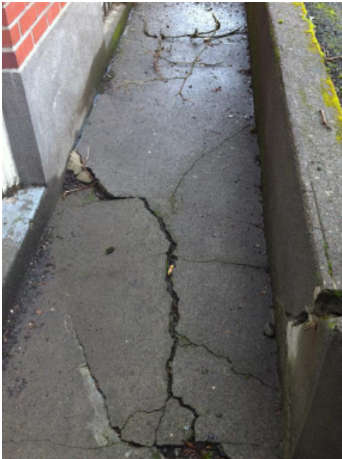
Damaged concrete slab outside Door X007
