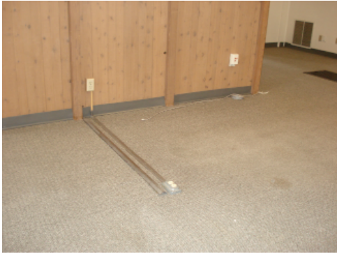
Electrical to be removed at base of mezzanine stair
