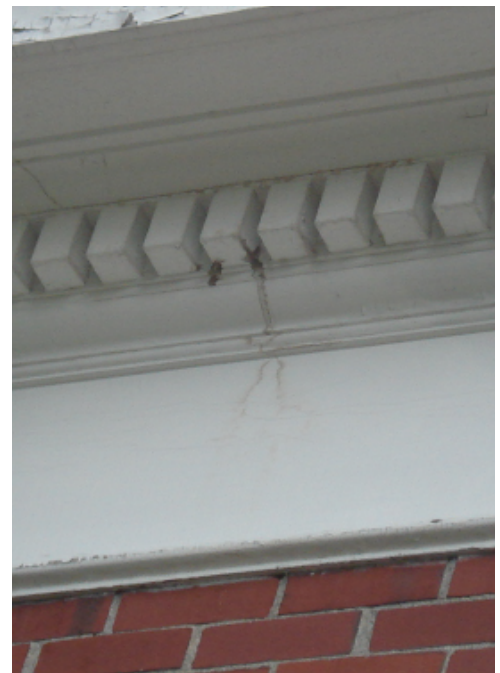
Water intrusion at dentils, underside of integral gutter
