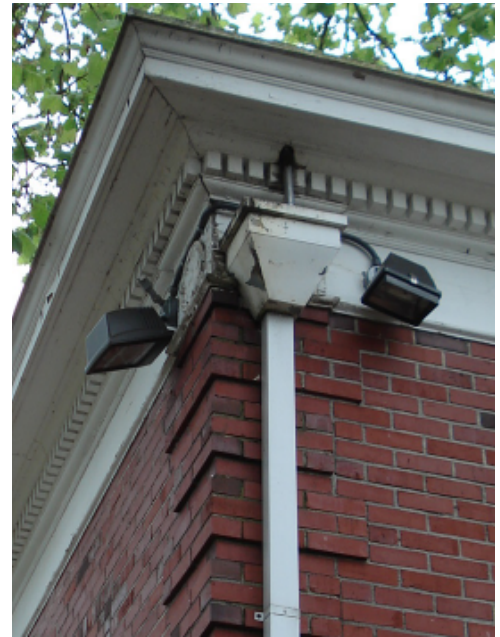
Scupper northeast corner of kitchen wing.
