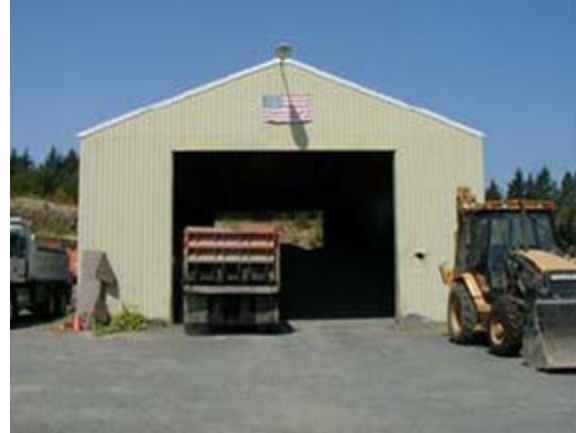
Road shop equipment Source: County Building & Property Data
