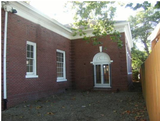
Northeast corner courtyard.
