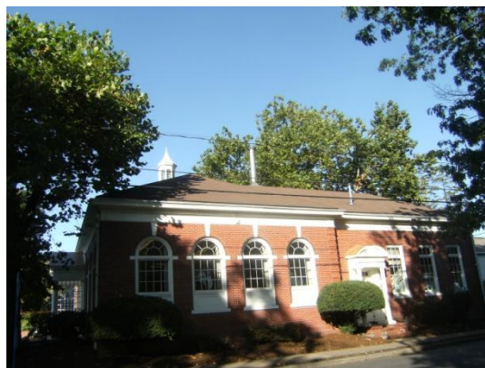
South building façade.
