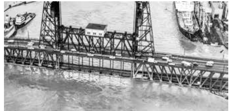
Photo source: Oregon Department of Transportation
