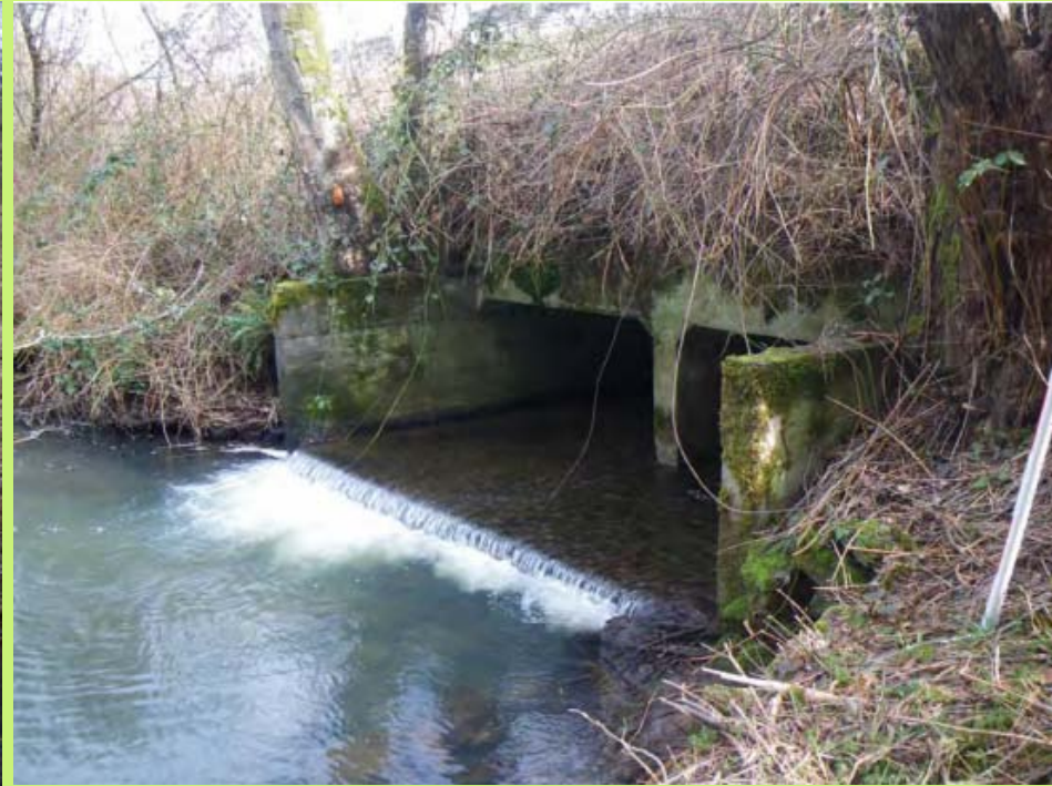
Outlet of Culvert
