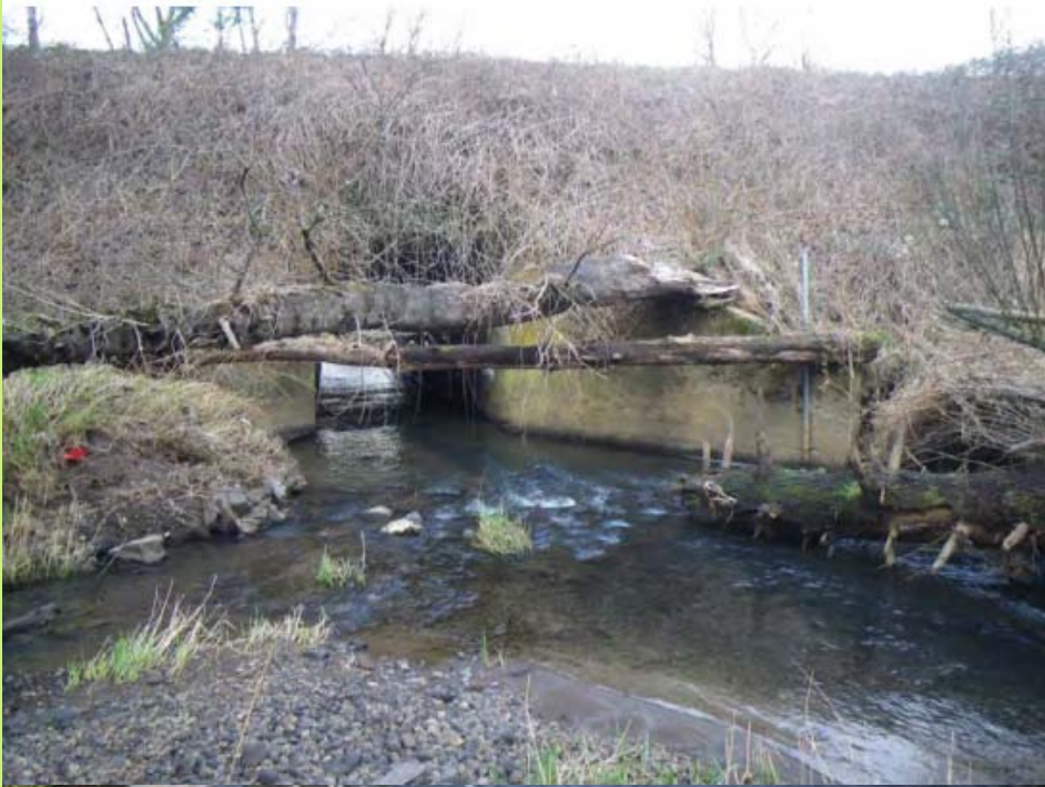
Inlet of Culvert
