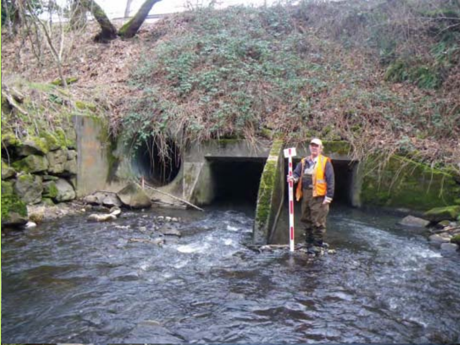
Inlet of Culvert
