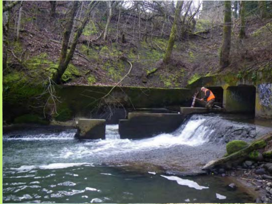
Outlet of Culvert
