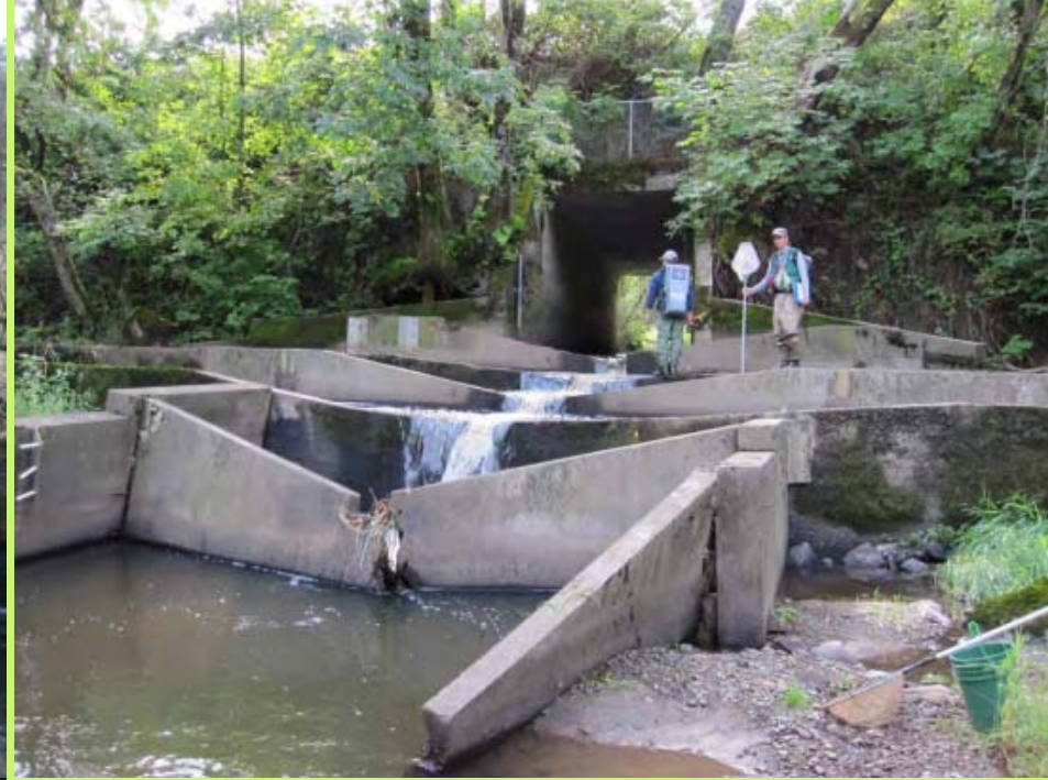
Outlet of Culvert
