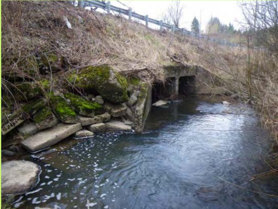
Inlet of Culvert
