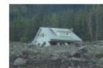
channelized debris flow
