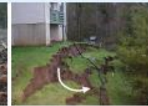
translational slide (most slides are combinations of translational and rotational movement)
