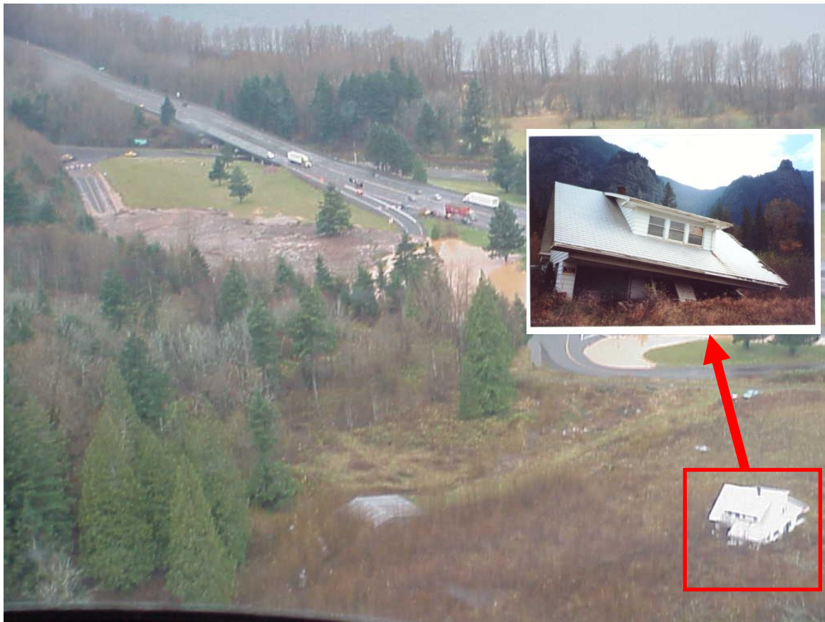
Figure 3.3-3 Landslide along Interstate 84 in the Dodson-Warrendale Area, December 2, 2001
