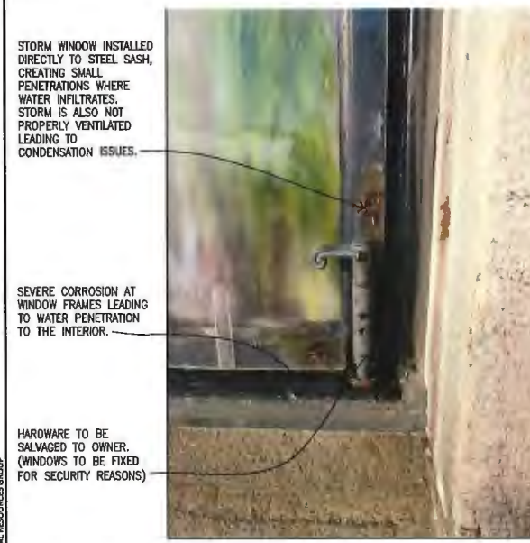
10 BALCONY WINDOW - EXISTING CONDITION NTS
