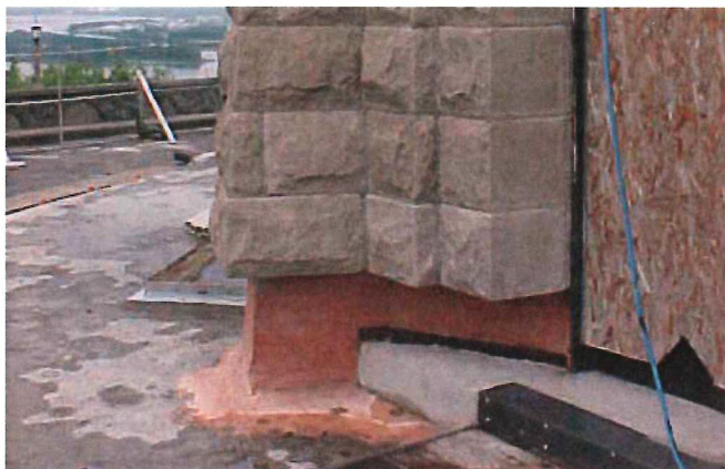
Base stone being replaced
