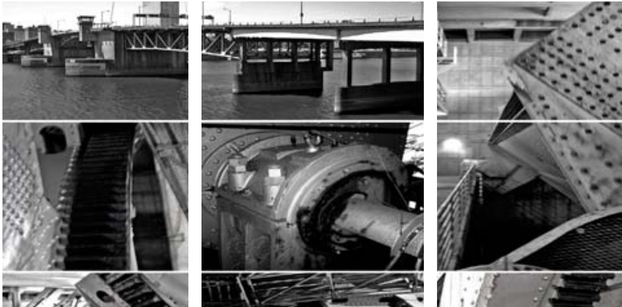
Photo Credit: Morrison Bridge by Jeff Kubina
