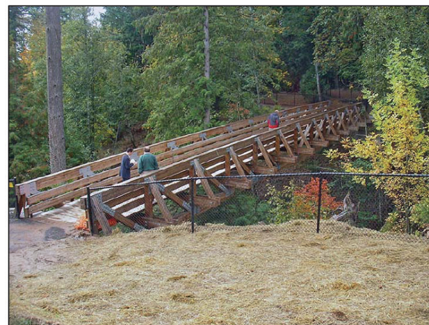
4 EXAMPLE: PONY TRUSS BRIDGE SECTION
