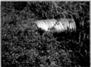
SE 146 Ave connector path to Springwater Corridor (southwest of Powell Butte) right after installation - water in swale next to rail berm and trail flows through corrugated metal pipe, vegetation will grow and obscure pipe
