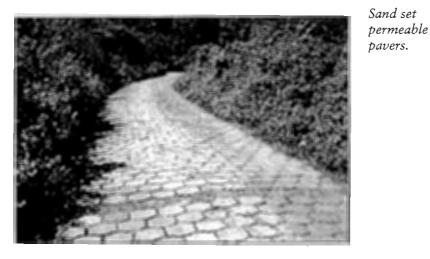
paving units are held in place by countersinking them into the trail bed so that their surfaces are flush with the surface of the surrounding undisturbed soil. Grade and curves are limitations. Some sources recommend that permeable pavers be restricted to slopes no greater than 5 percent. Some types of permeable pavers are favored for trails in water resource protection areas because of their ability to infiltrate precipitation.
