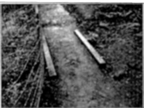
Woods Memorial Park - biking path (under construction), intercepting runoff in swale and piping under segment of causeway in poorly drained area near Woods Creek
