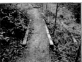
Woods Memorial Park - causeway using 4" x 6" timbers (under construction with temporary metal fence to protect new plantings and prevent trampling of bank of Woods Creek)
