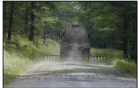
Figure 4. Spray application of topical dust suppressants.
