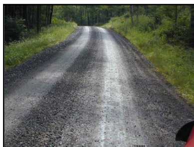
Figure 13a. Photographs of sites 1 day after dust suppressant application.
