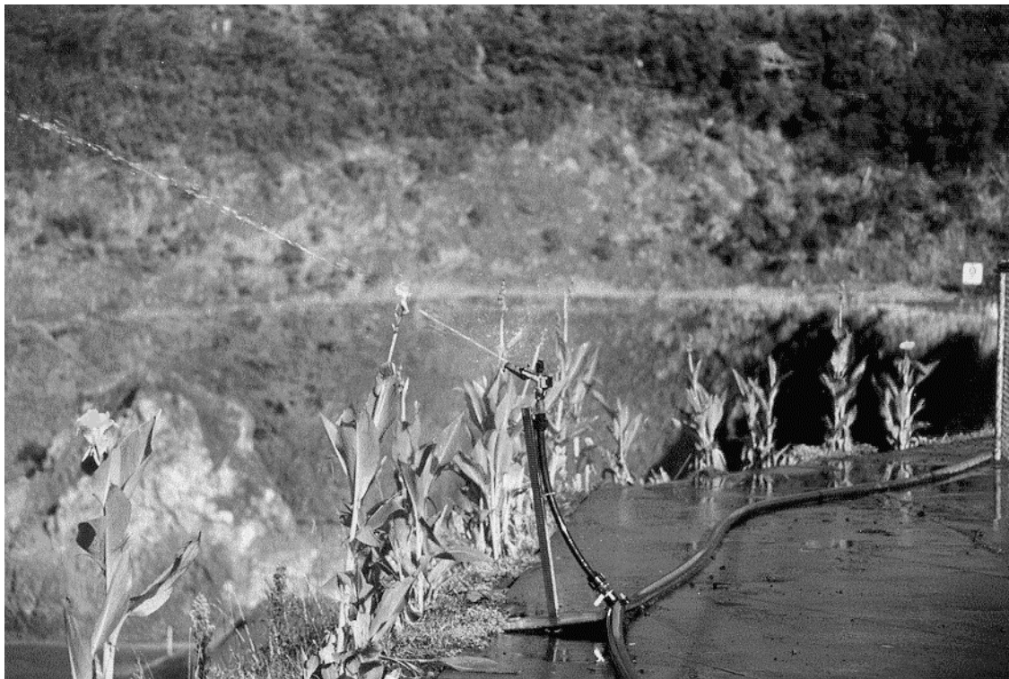
Figure 4: Wet suppression is an important dust control method for unconsolidated material, stockpiles and unpaved surfaces
