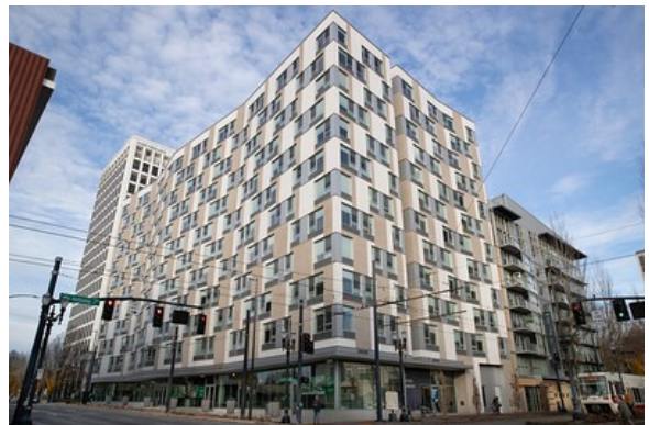
The Louisa Flowers, a recently built affordable apartment building, MultCo Communications
