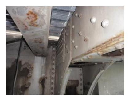
Rusted structural steel supporting the bridge deck will be repainted.
