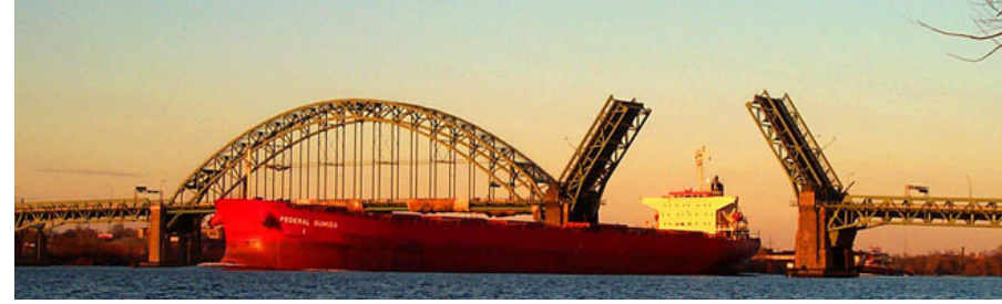
Tacony-Palmyra Bridge, Pennsylvania
