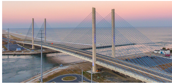
Indian River Inlet Bridge, Delaware
