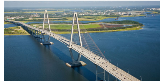
Copper River Bridge
