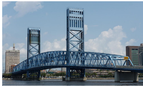
Main Street Bridge, Florida
