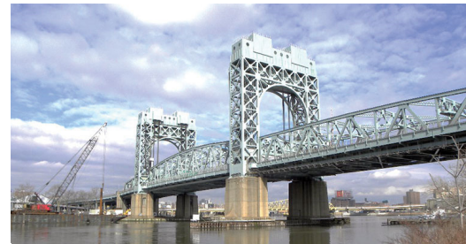
Triboro (Harlem River) Bridge
