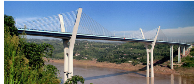
Chongqing Expressway Bridge
