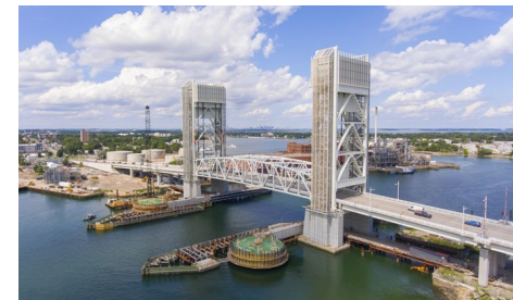
Fore River Bridge
