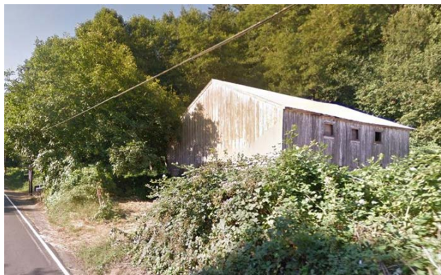
Figure 4: Existing Agricultural Building
