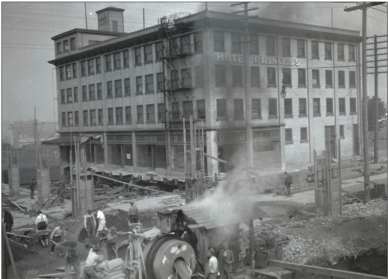
Figure 5-7. The Princess Hotel at NE 3rd and Burnside relocated north for construction of the new Burnside Bridge in 1925.
