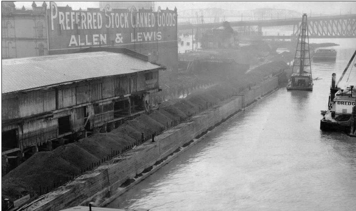
Figure 5-28. Remaining dock and Harbor Wall construction with placement of fill at the Allen & Lewis warehouse, looking downriver. Note the Gillen-Cole building is gone and the Portland Gas Manufacturing Purifying House to the north is partially razed. Compare with Figure 5-29. Photo dates December 23, 1928.
