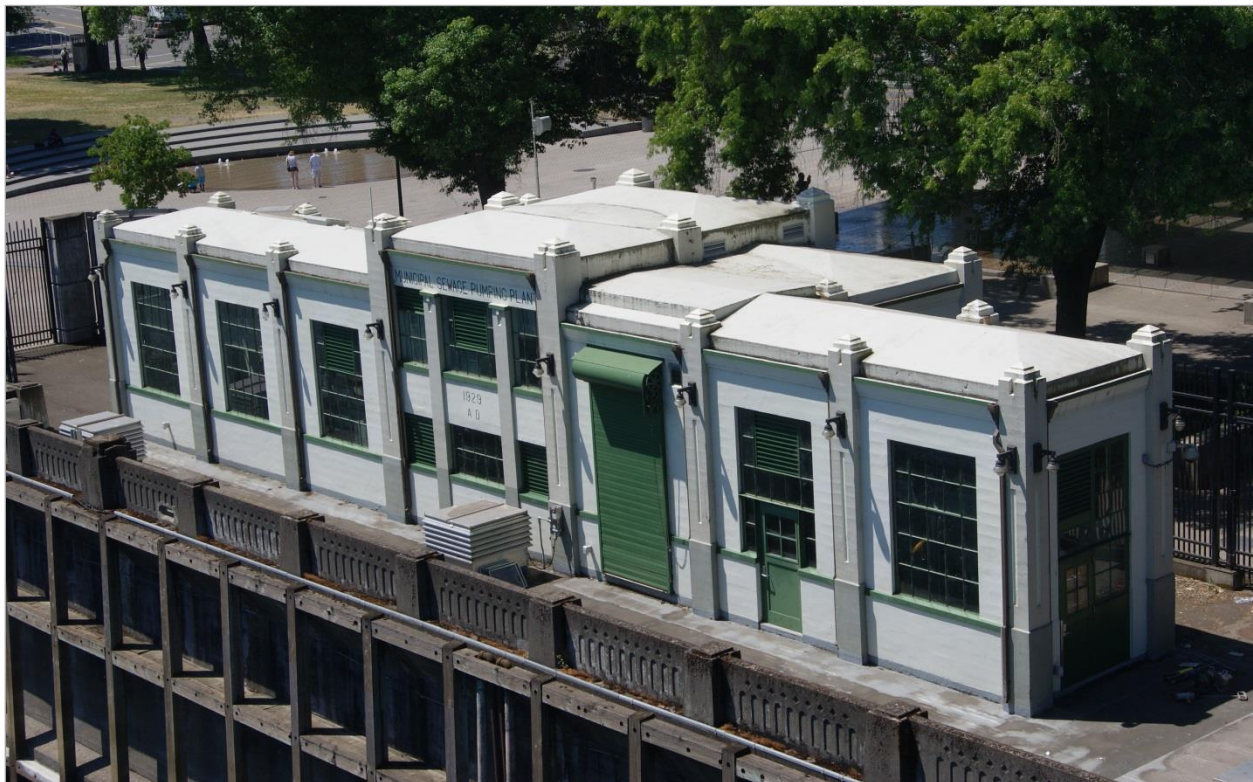
Figure 5-64. A view of the Ankeny Pump Station taken from the Burnside Bridge.
