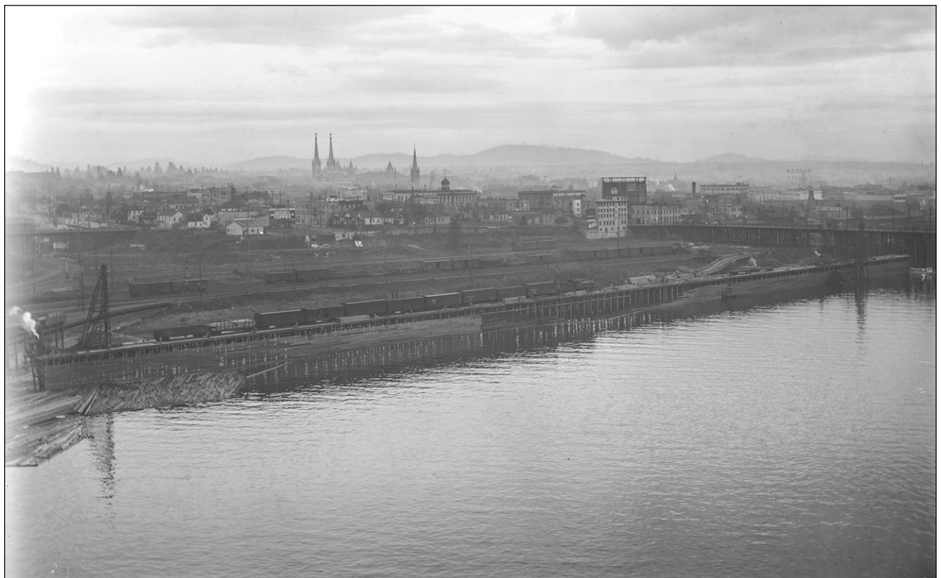
View: View of the historic railroad alignment (ca. 1918), view is to the east. The eastern approach of the original Burnside Bridge is on the right (Oregon Historical Society OrHi44795).
