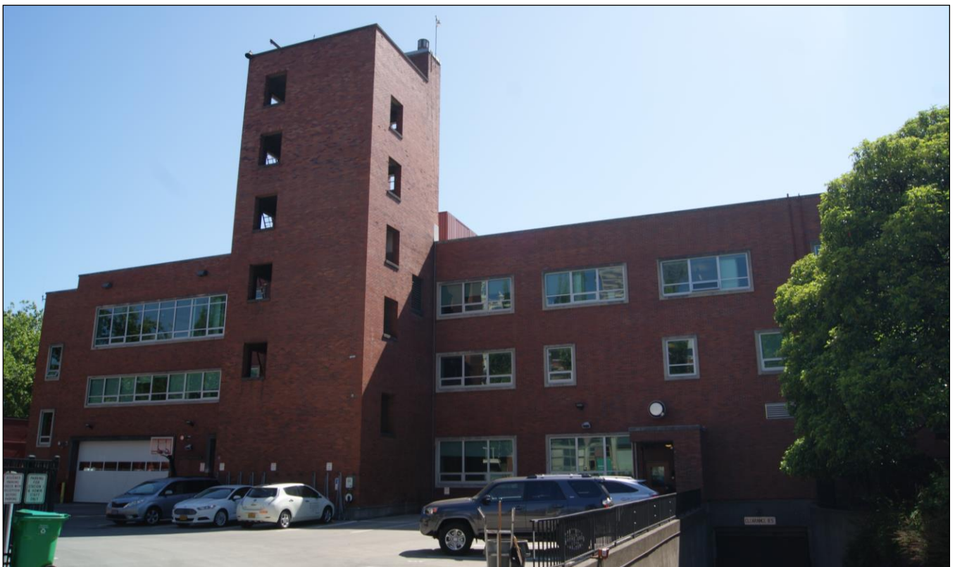
View: The rear (west) façade of the Central Fire Station. The view is towards the northeast.
