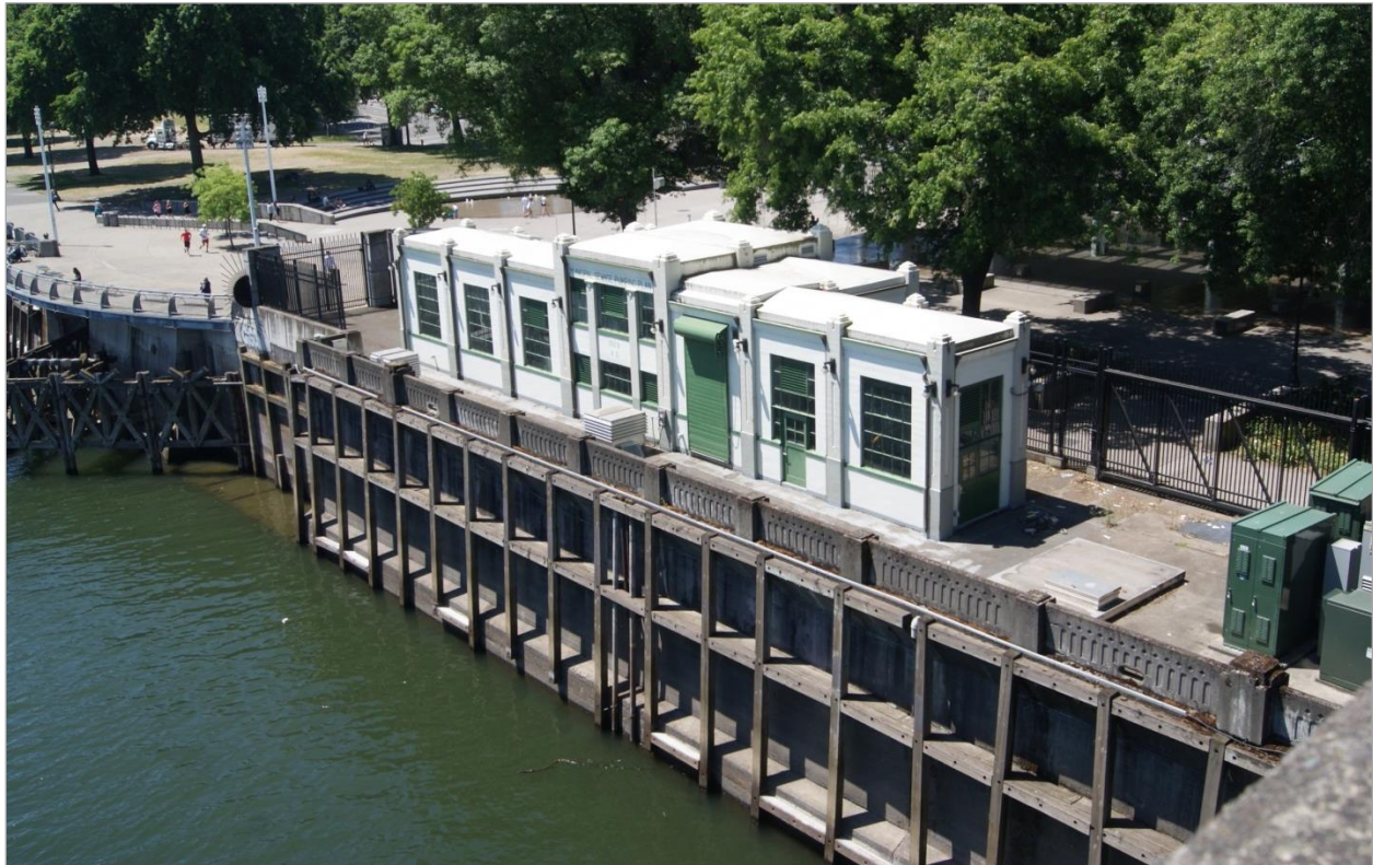
Figure 5-63. A view of the Portland Harbor Wall and the associated Ankeny Pump Station; the view is towards the southwest.
