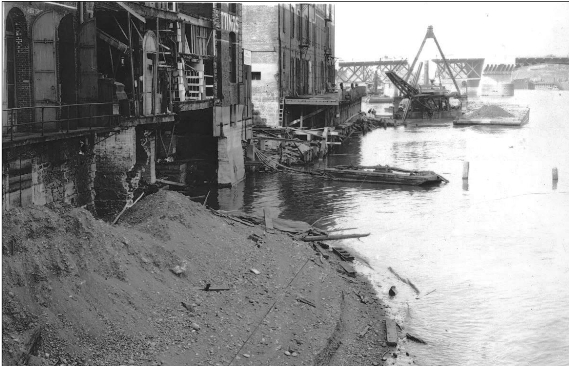
Figure 5-34. Dredging Harbor Wall fill, Burnside Bridge in the background. Photo dated April 26, 1928.
