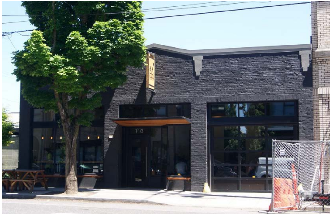
The building's west façade; the view is towards the east.
