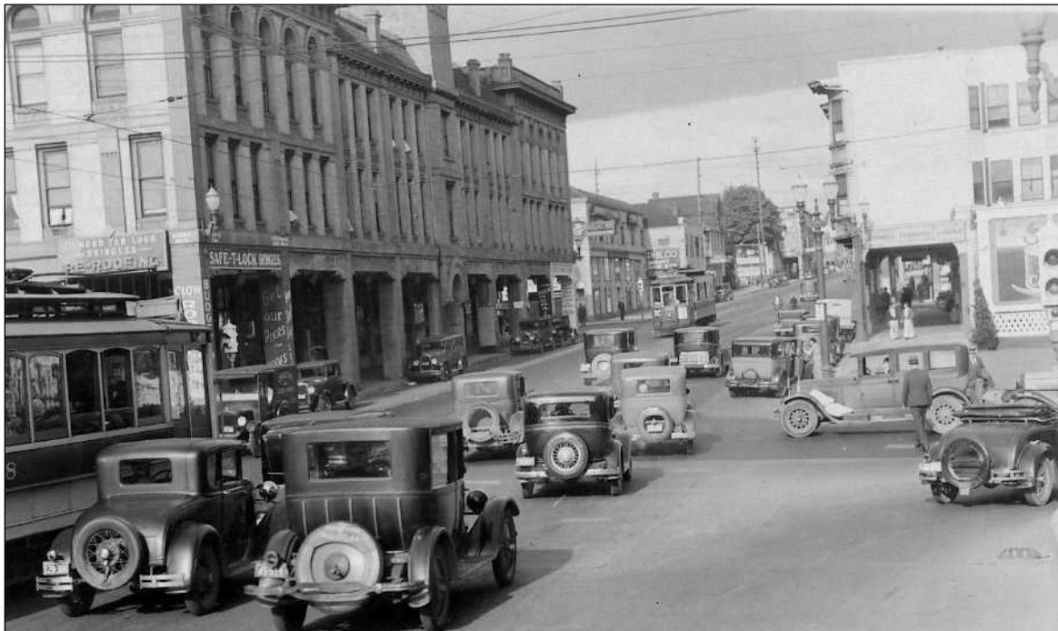
Figure 5-9. Looking east along E Burnside Street in 1933 from the east end of the Burnside Bridge showing arcades constructed to accommodate widening of E Burnside.
