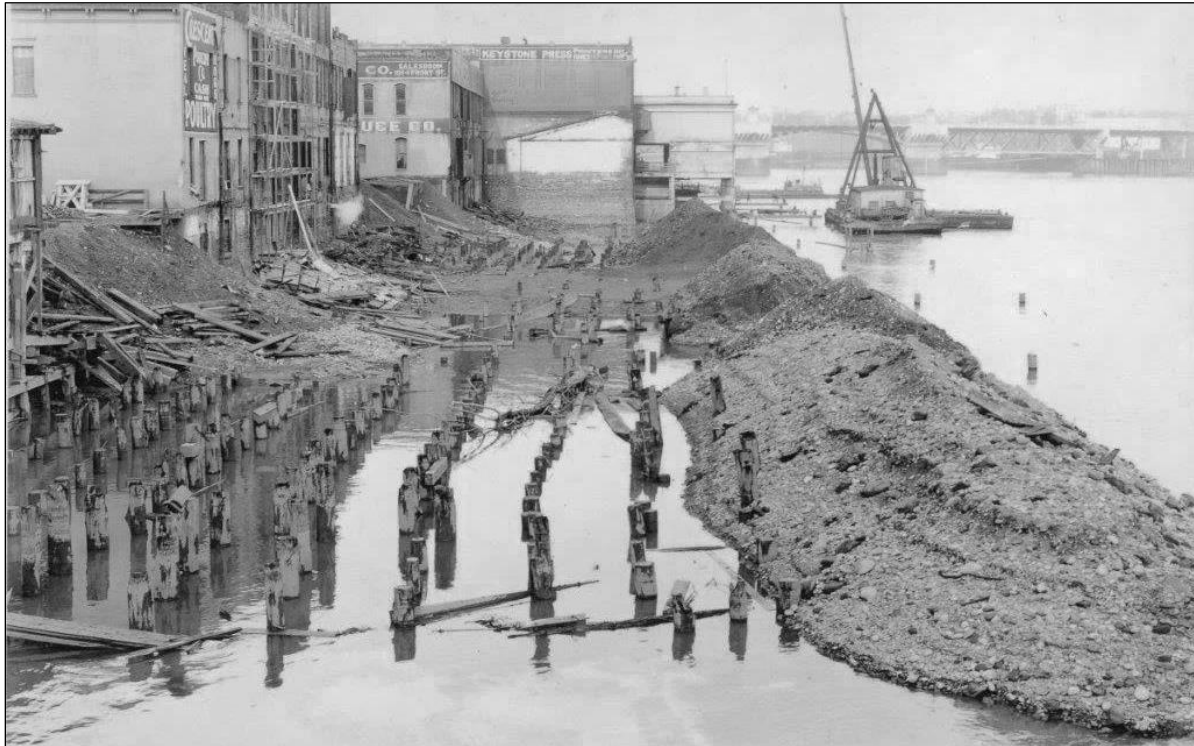
Figure 5-30. Remnant piling from demolished docks as Harbor Wall construction begins, looking downriver to the Burnside Bridge. Photo dated January 28, 1928.
