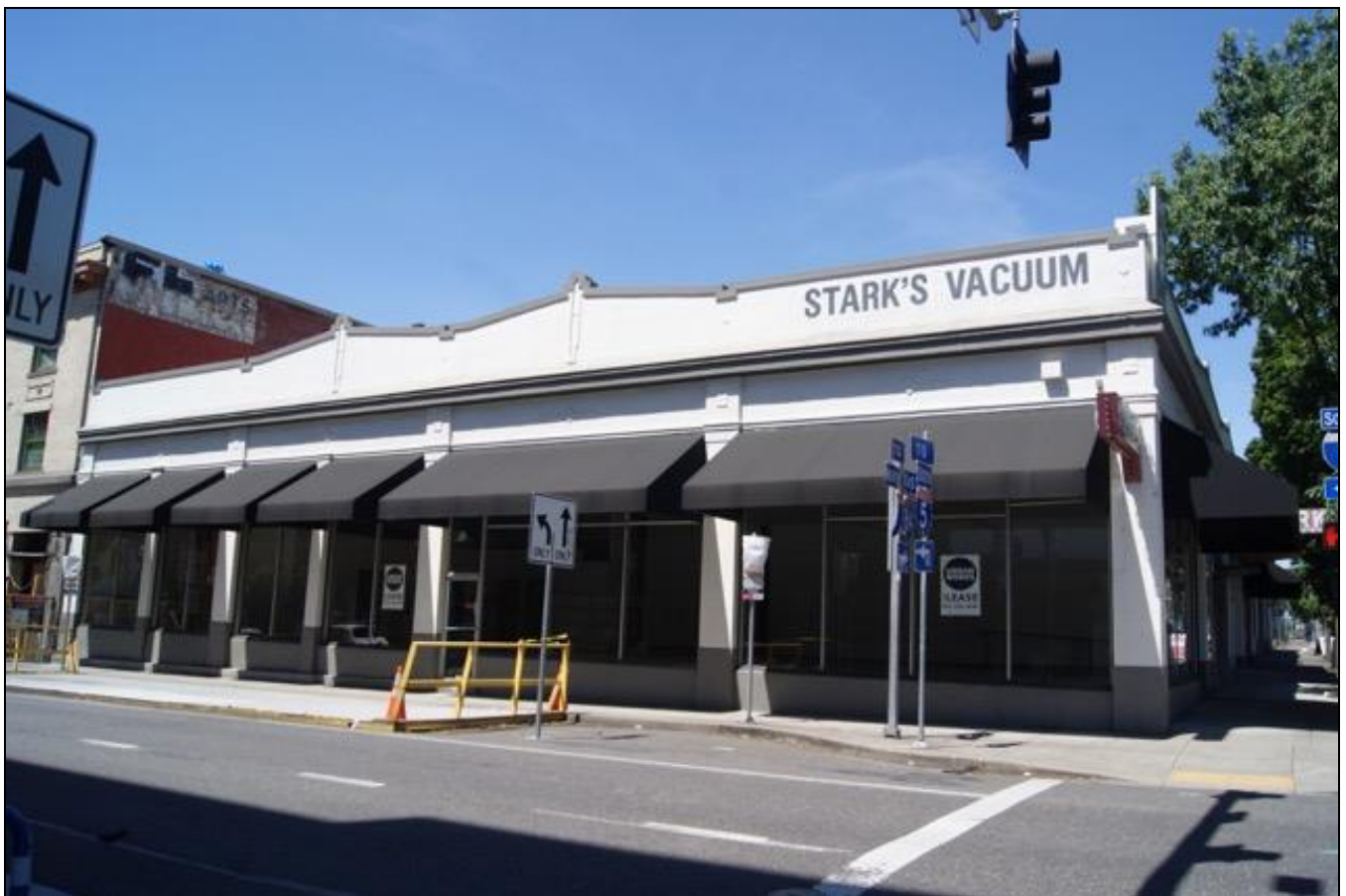
View: The south building segment (1926) showing the south façade; the view is to the north-northwest.
