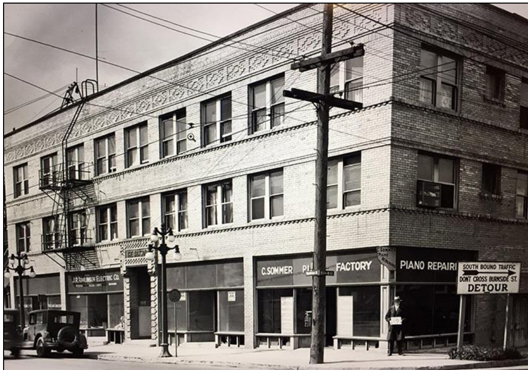
A historic photo of the Jackson Apartments showing the commercial storefronts that faced Union Avenue (NE Martin Luther King Blvd.) The view is towards the southwest. (Photo from www.unionarmspdx.com ).
