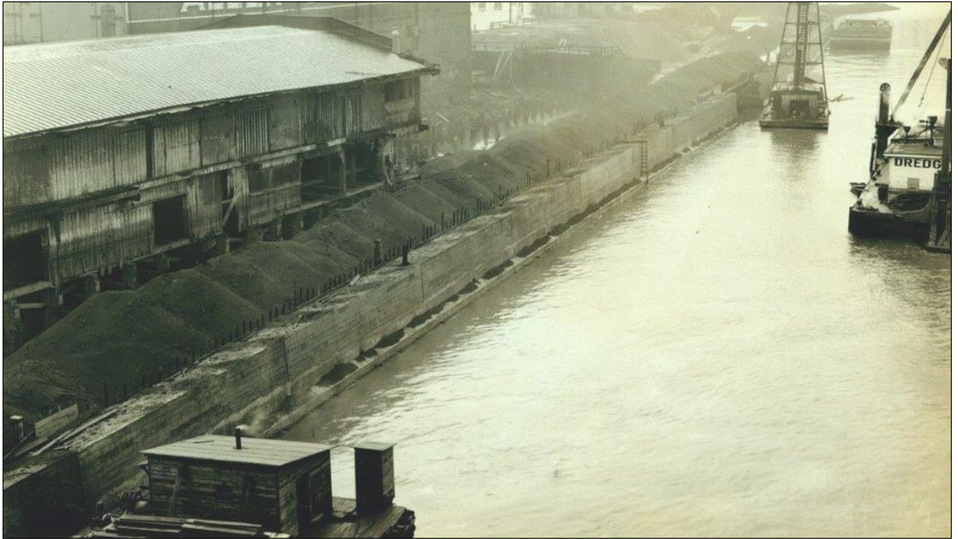
View: Portland Harbor Wall under construction in 1928, view facing northwest.
