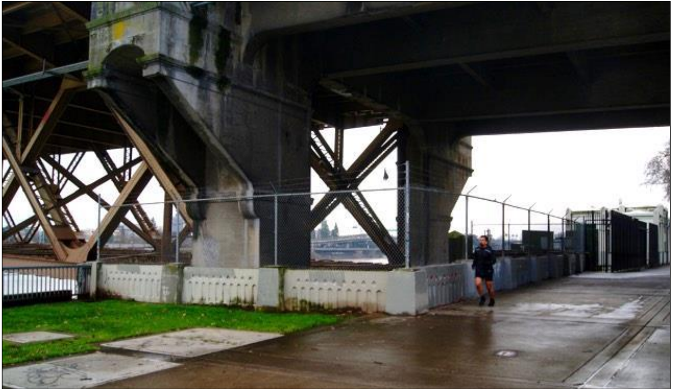
View: The Harbor Wall where it is built around Pier 1 of the Burnside Bridge, view facing southeast.
