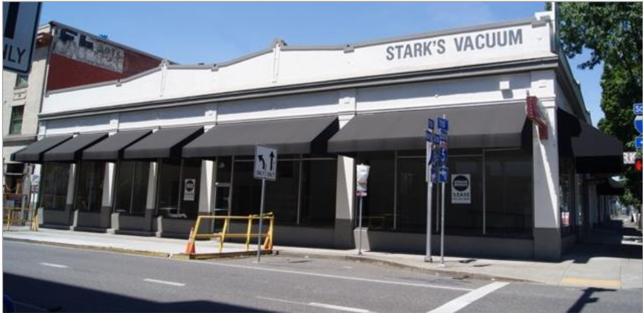
Figure 5-67. The Stark’s Vacuum Building facing NE Couch Street.
