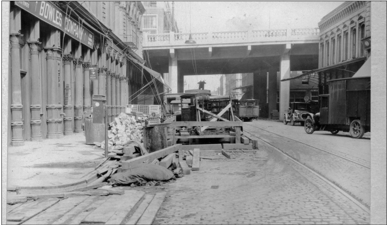
Figure 5-24. Open trench construction of the Front Street intercepting sewer along Front Street, looking north to the Burnside Bridge approach. Photo dated 1928.
