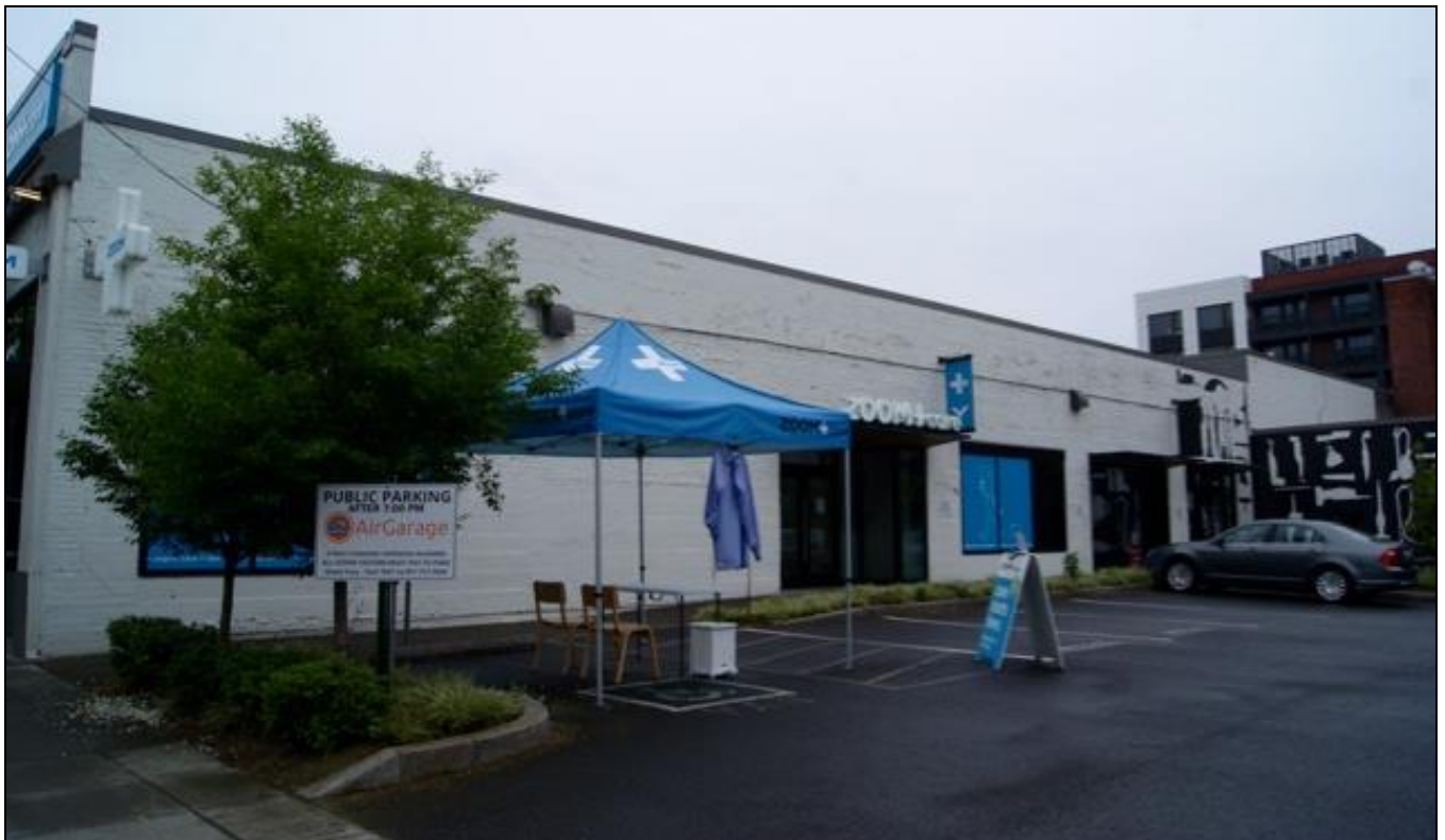
View: The north building segment's west façade; the view is towards the southeast.
