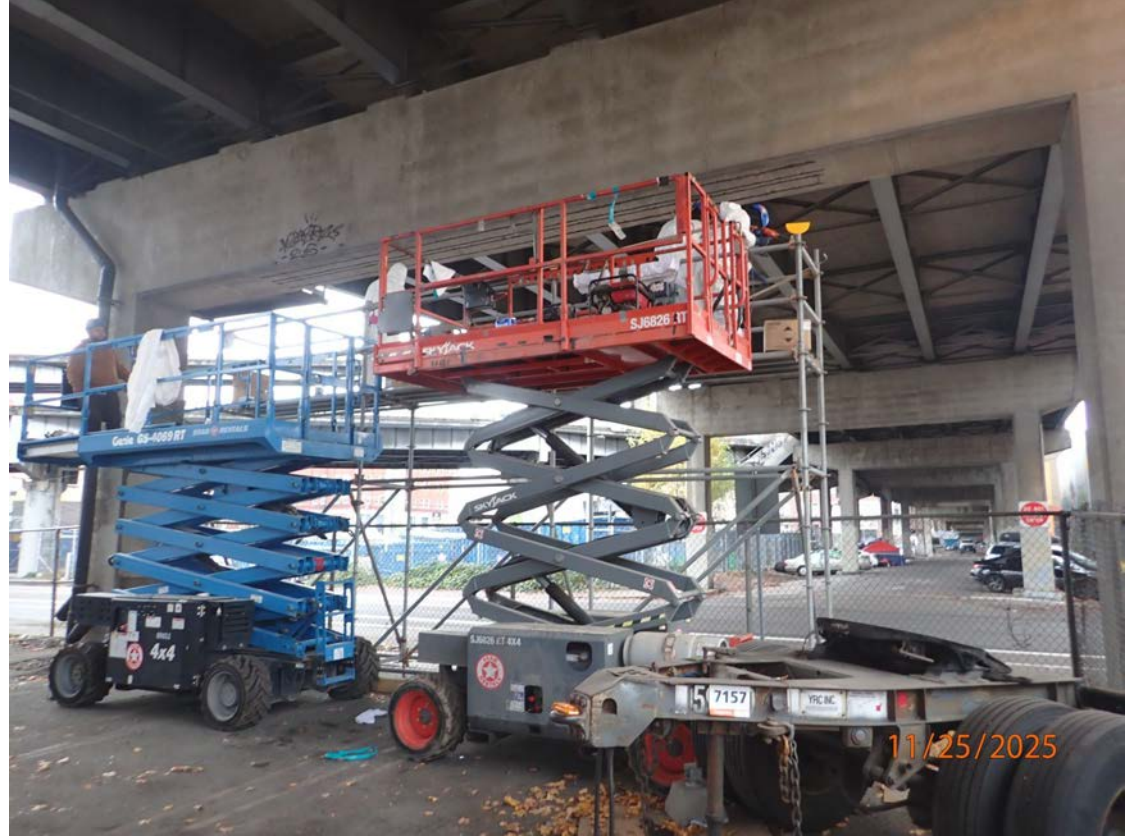
Installation of titanium bars to increase the strength of the beam
