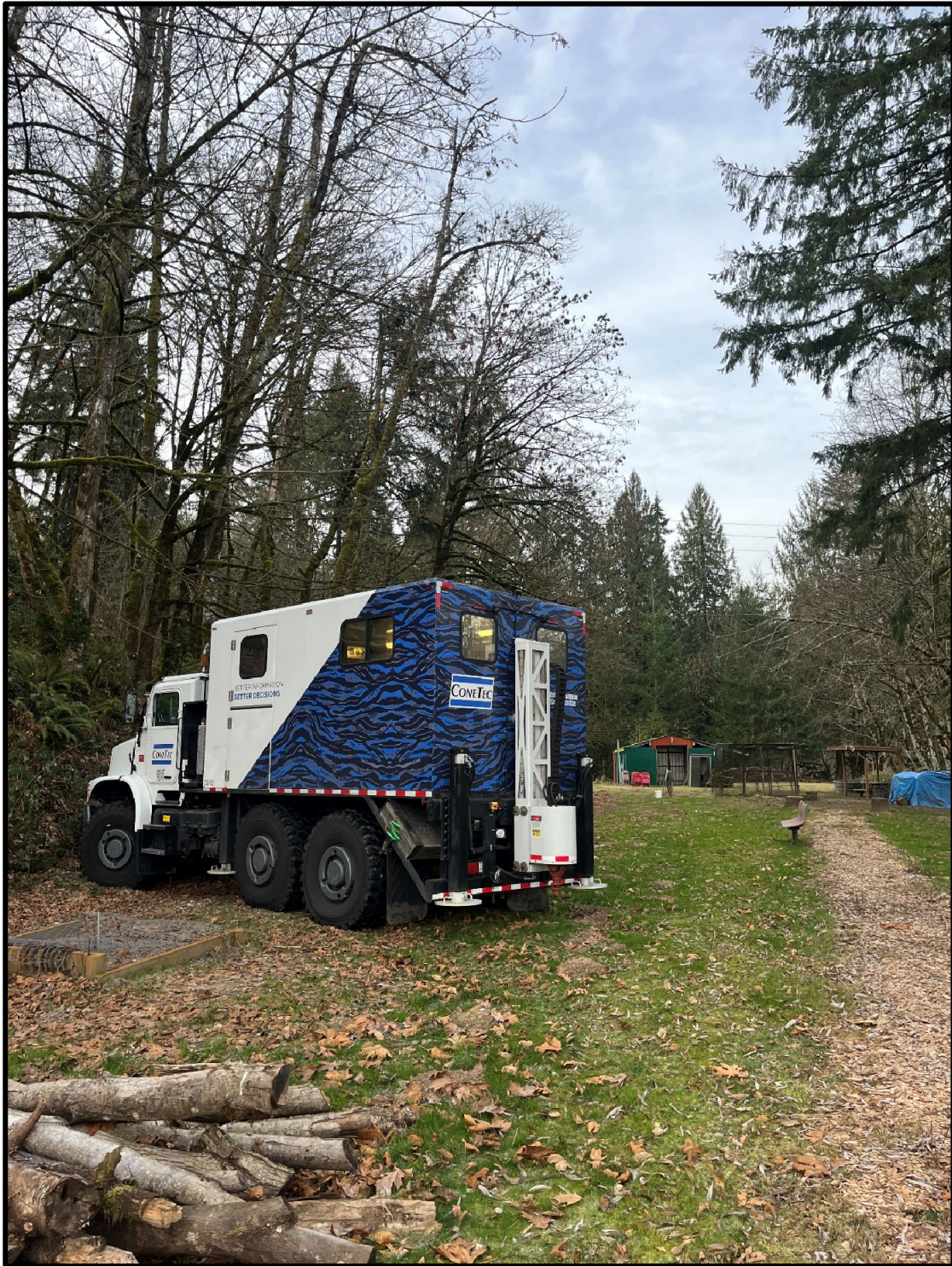
Performing CPT-2, Facing South
