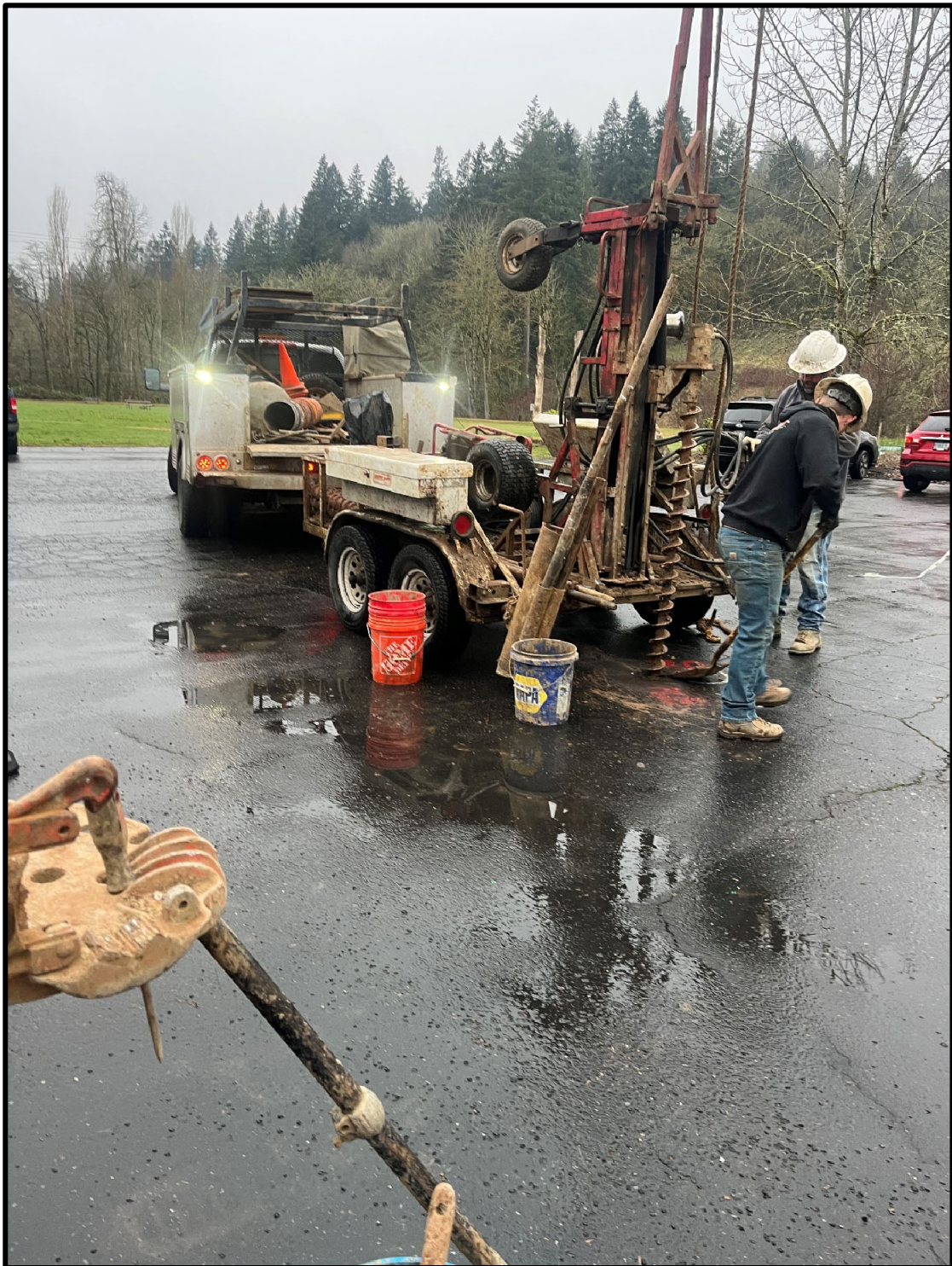
Drilling SB-1, Facing Southwest
