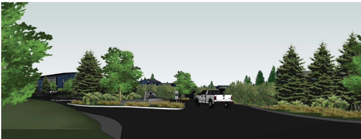
Figure 19: View from the Filtration Facility Front Entry
