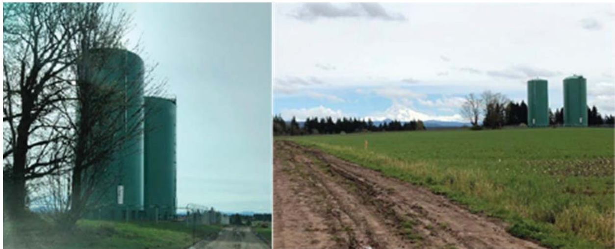
Figure 12: PHWD Water Tanks (35524 Carpenter Lane)
