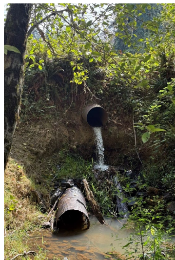
Figure 2. Earth-fill dam is a fish passage barrier
