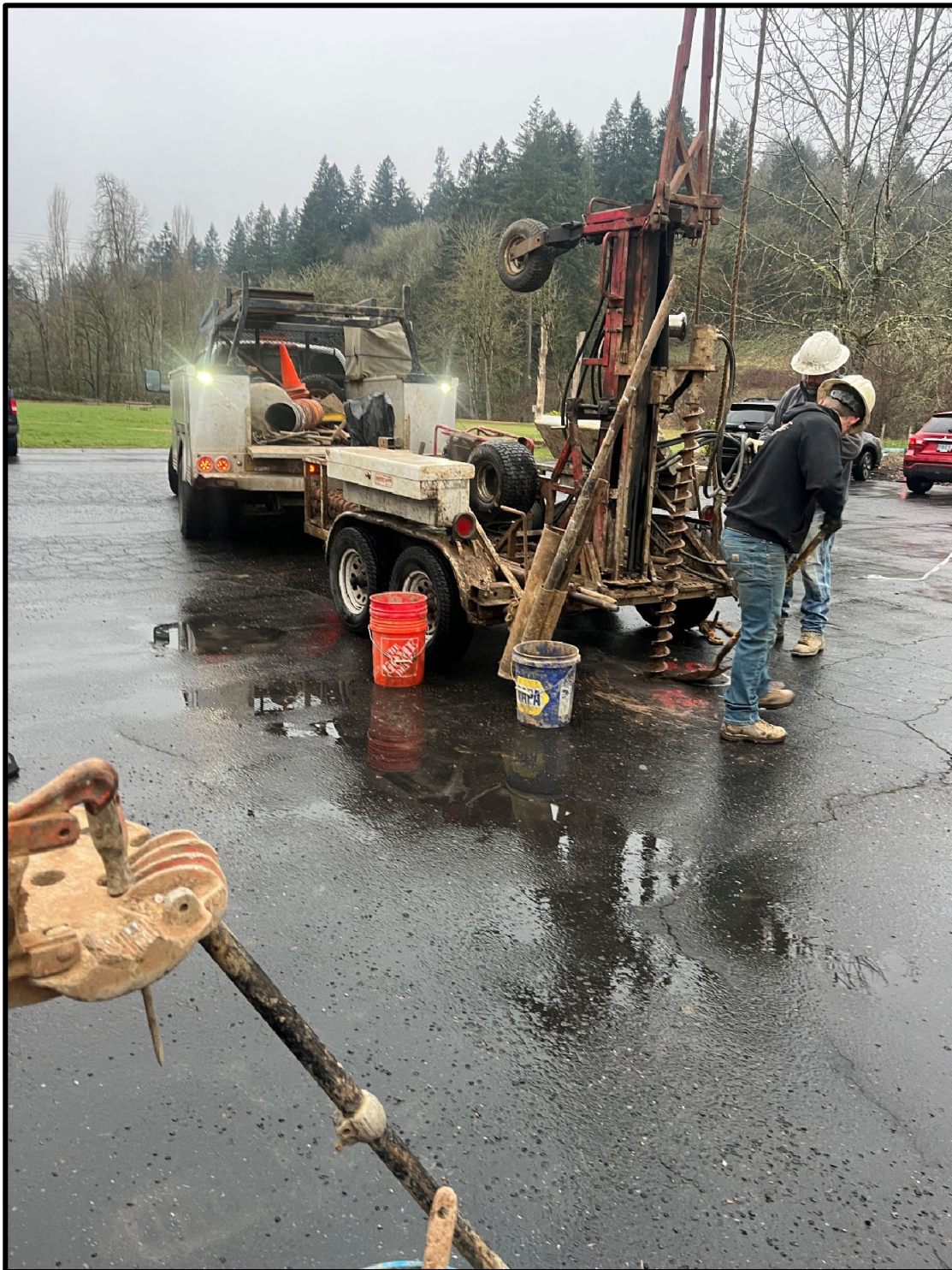
Drilling SB-1, Facing Southwest
