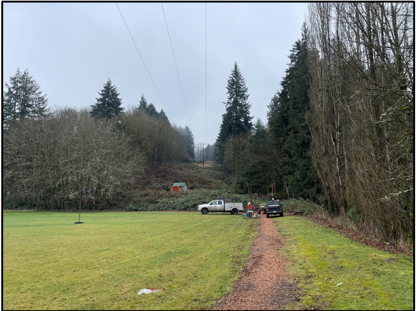
Drilling SB-3, Facing East
