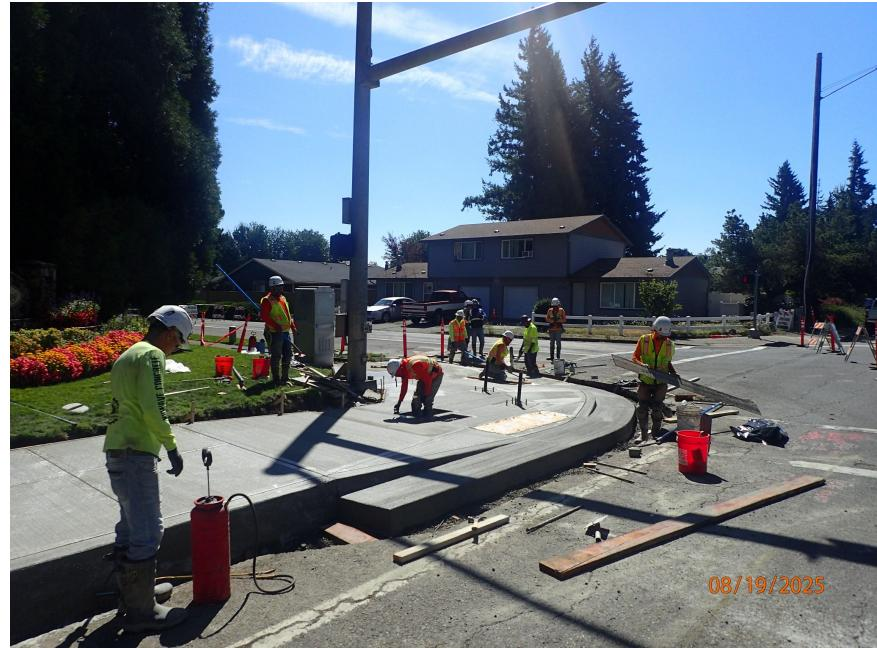
Photos taken by Inspector Phil Ledbury of Transportation Crew members constructing a sidewalks and curb ramps along SW 257th Drive, Troutdale (between Historic Columbia River Highway and SE Stark Street).
