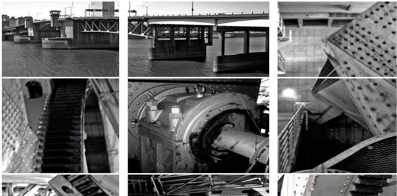
Photo Credit: Morrison Bridge by Jeff Kubina
