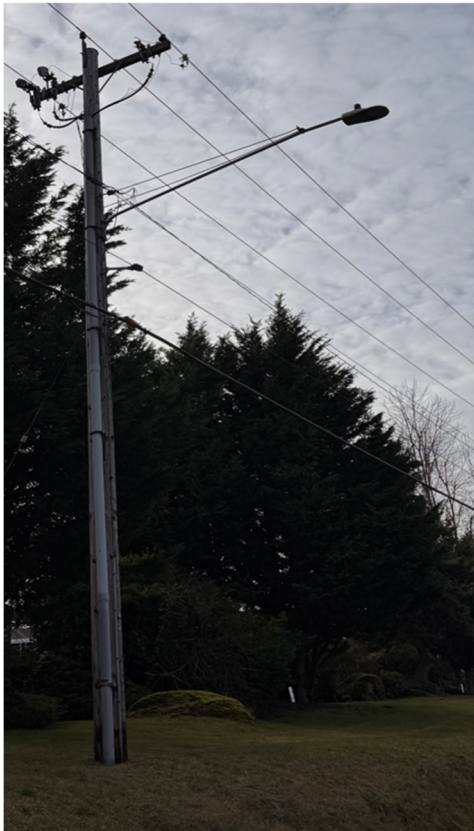
Figure 2: Cobra Head Style Luminaire Mounted on Wood Utility Pole
