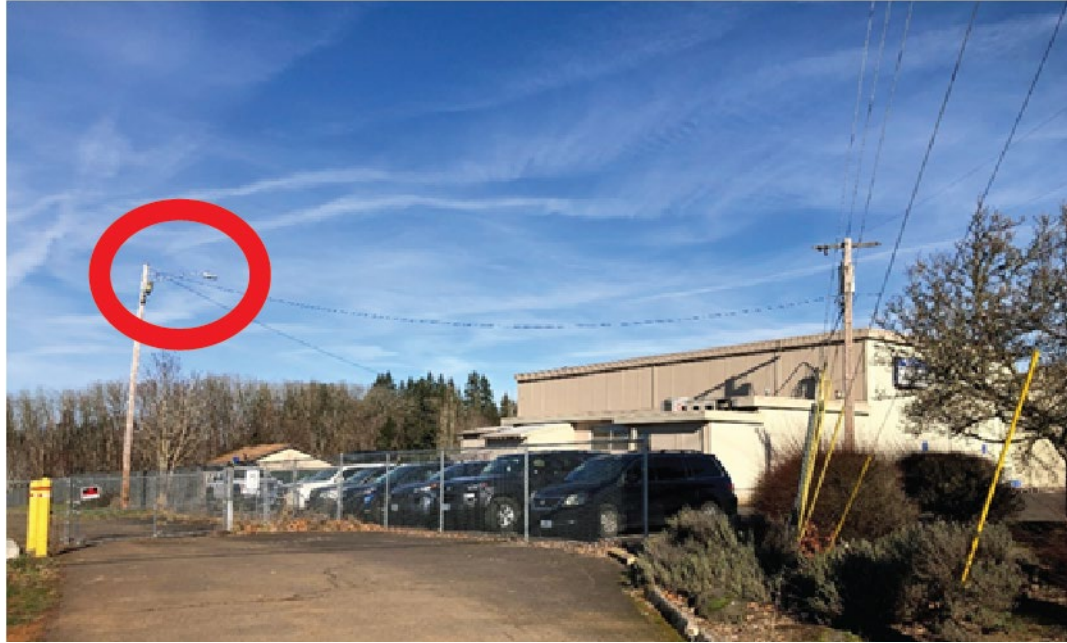
Figure 11. Oregon Trail Academy (Proctor Road)—Unshielded Pole Lights for Building and Parking Area
