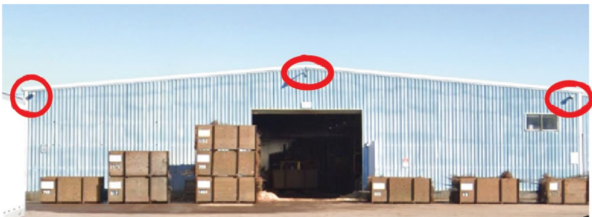
Figure 9. J. Frank Schmidt Company Unshielded Wall Lighting (327 th Avenue)
