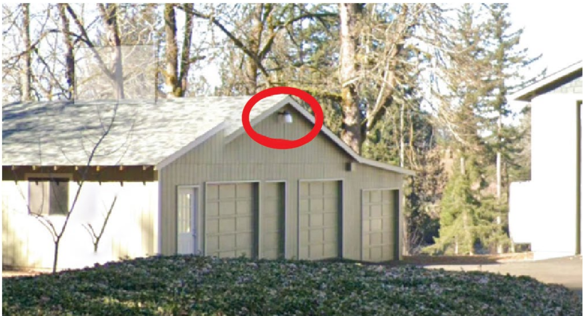
Figure 2. Unshielded Wall Lights Illuminating Garage and Accessory Structure Parking Areas
