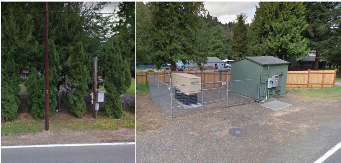
Figures 1 and 2. Existing pole-mounted CPRs and utility structures along Lusted Road
