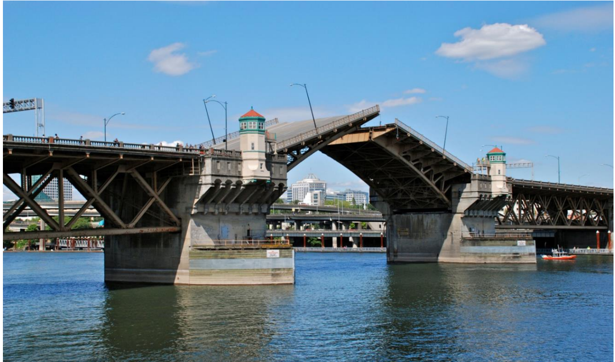
Figure 1. Burnside Bridge Main River Span Bridge over the Willamette River, Portland, Oregon
