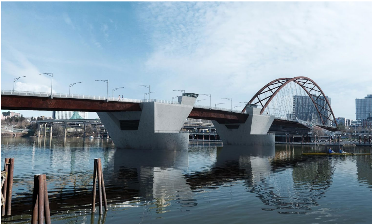
with Tied Arch for eastside long span
