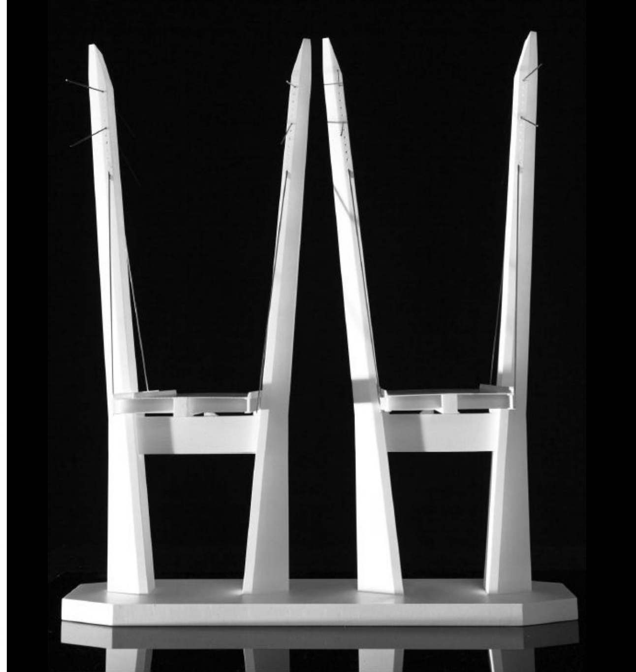
Component shaping – vertical tapering (migrating seams) make a significant difference to the visual form
