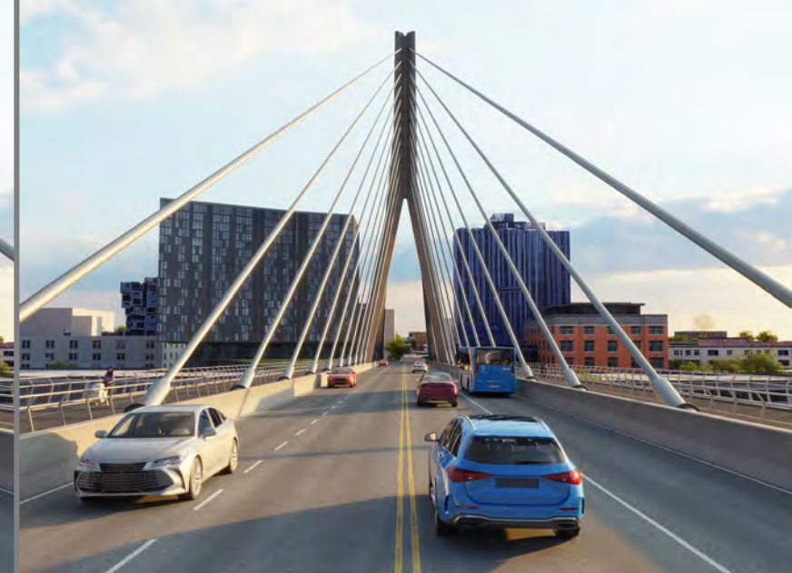
CS3- Inverted-Y tower
