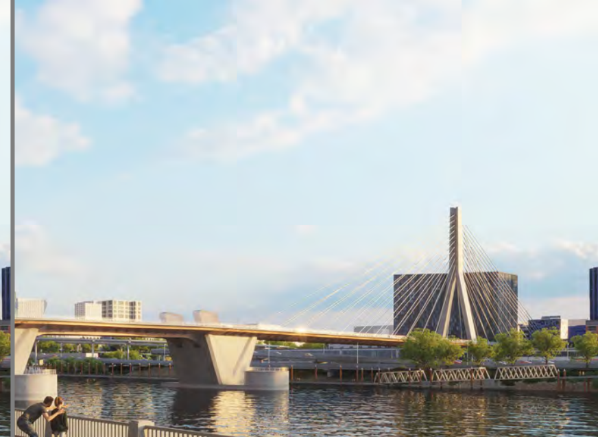
CS3- Inverted-Y tower
