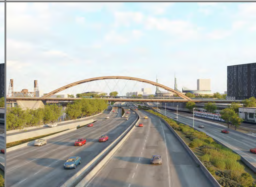
TA3- Braced vertical arches
