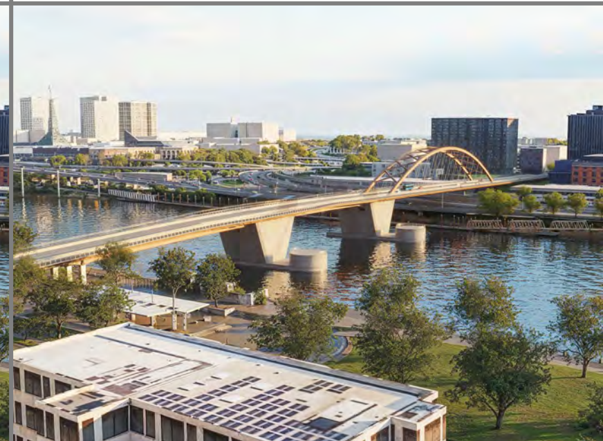
TA3- Braced vertical arches
