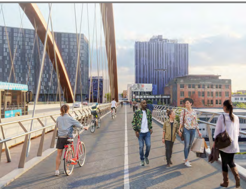
TA1-Unbraced vertical arches
