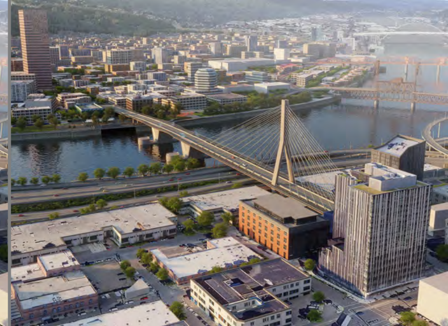
CS3- Inverted-Y tower
