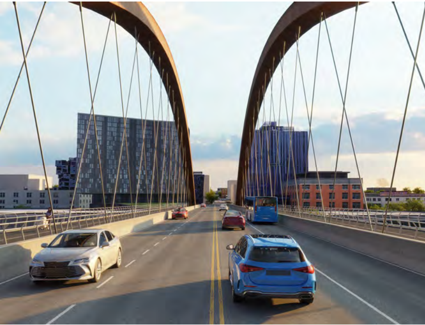
TA1-Unbraced vertical arches
