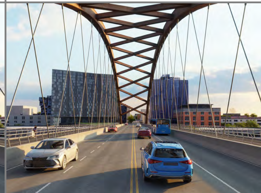
TA3- Braced vertical arches
