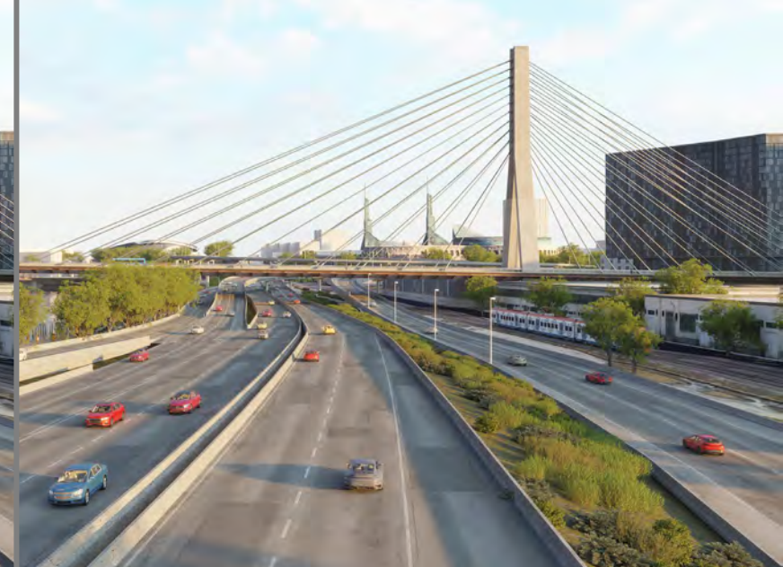
CS3- Inverted-Y tower
