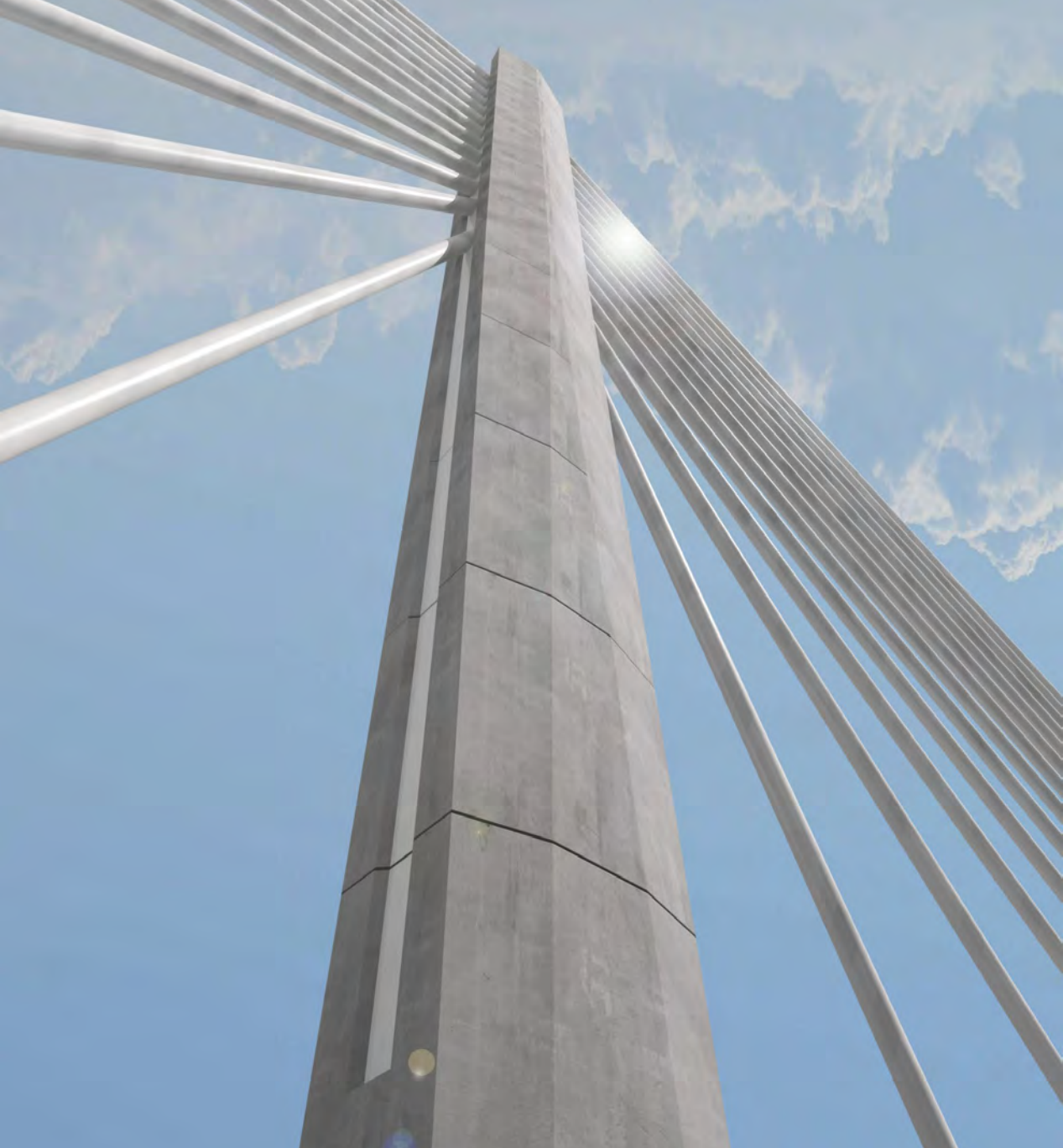
Component shaping – faceted forms make a significant difference to the perceived slenderness
