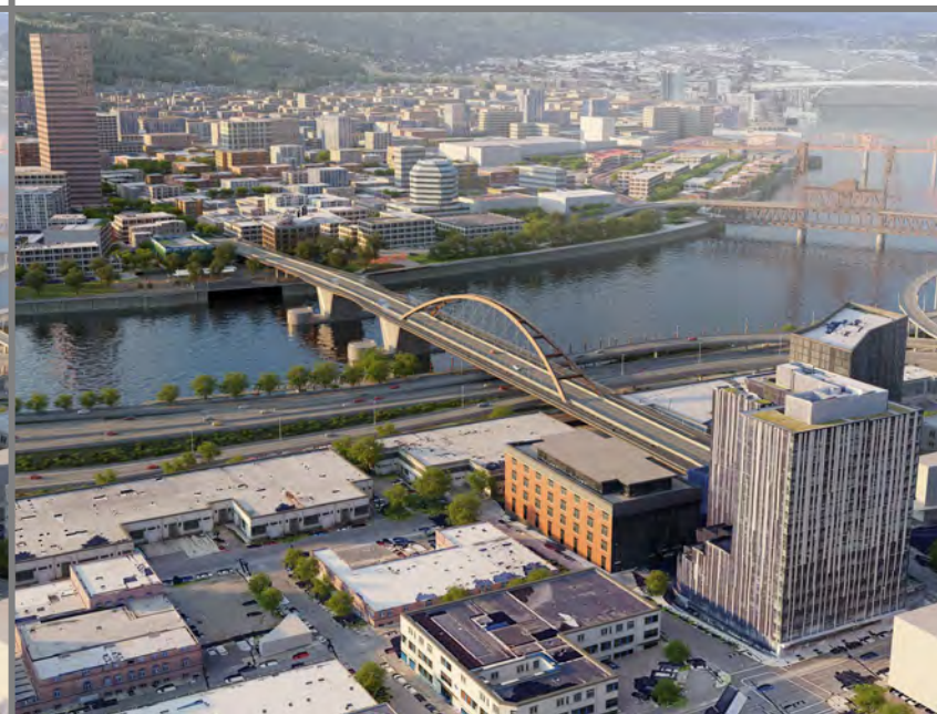
TA2-Braced basket-handle arch
