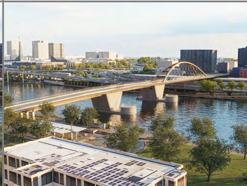
TA2-Braced basket-handle arch
