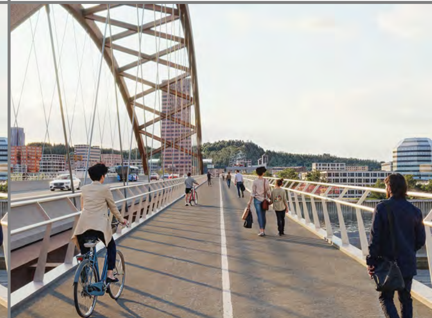
TA3- Braced vertical arches
