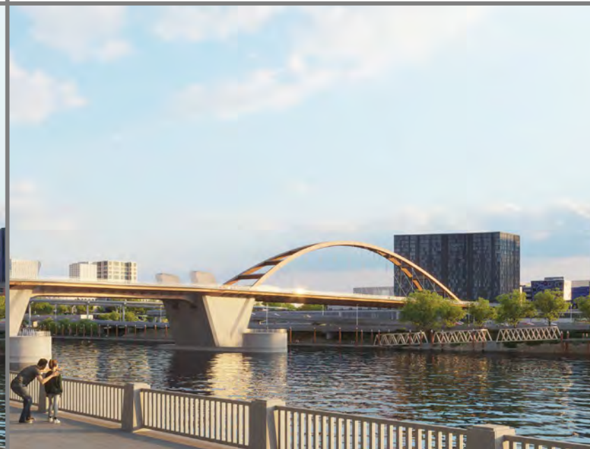
TA2-Braced basket-handle arch
