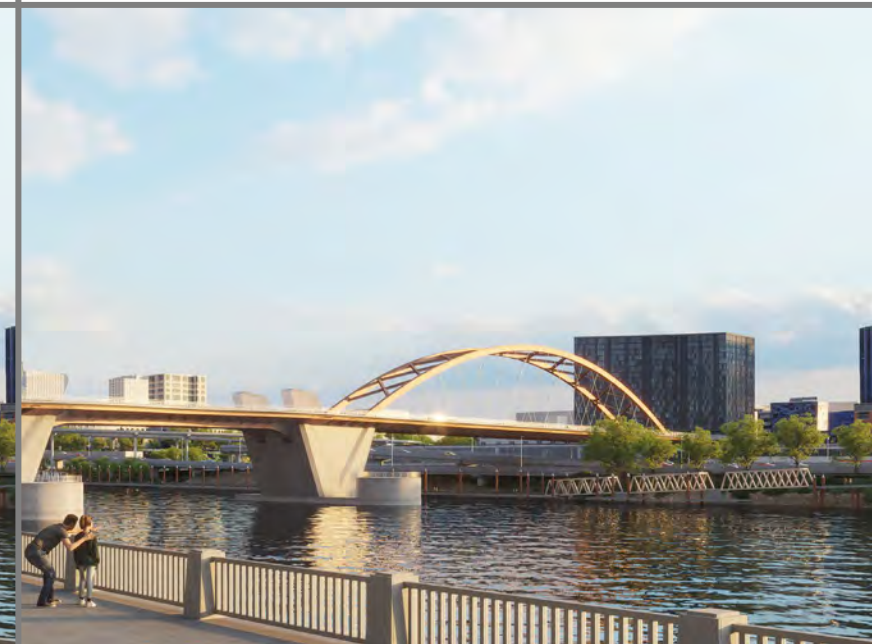
TA3- Braced vertical arches
