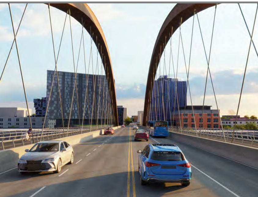
TA1-Unbraced vertical arches
