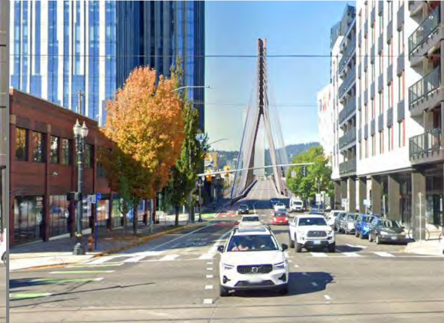
CS3- Inverted-Y tower
