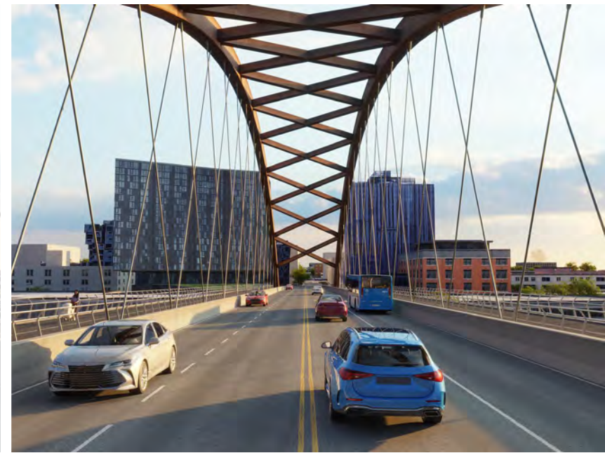
TA3- Braced vertical arches
