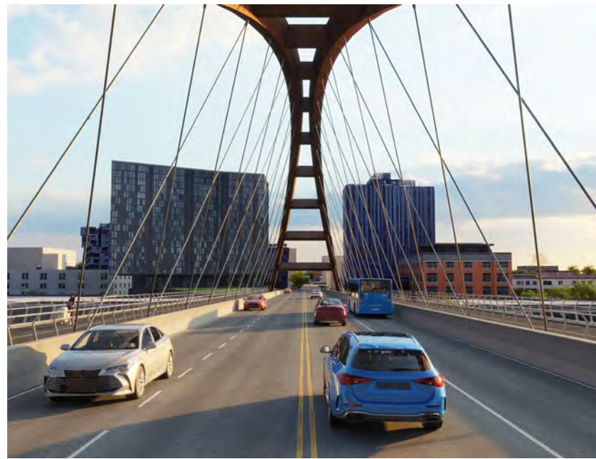
TA2-Braced basket-handle arch
