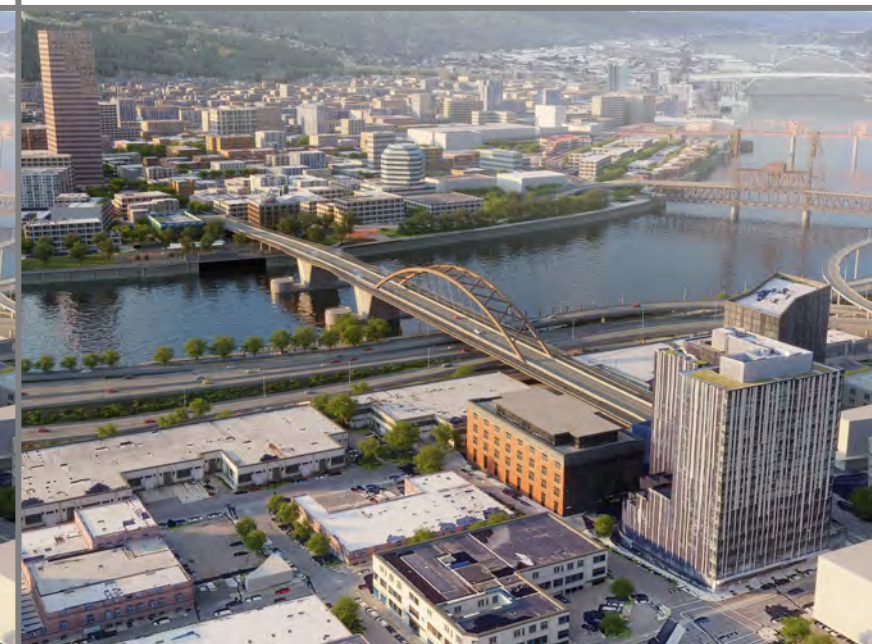
TA3- Braced vertical arches
