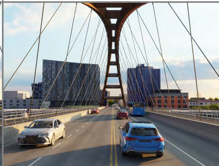
TA2-Braced basket-handle arch
