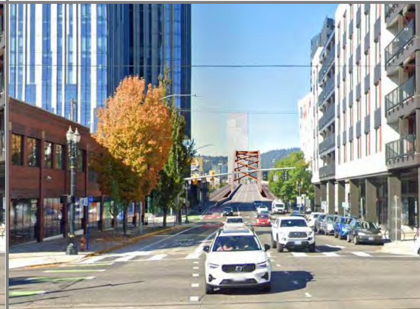
TA3- Braced vertical arches
