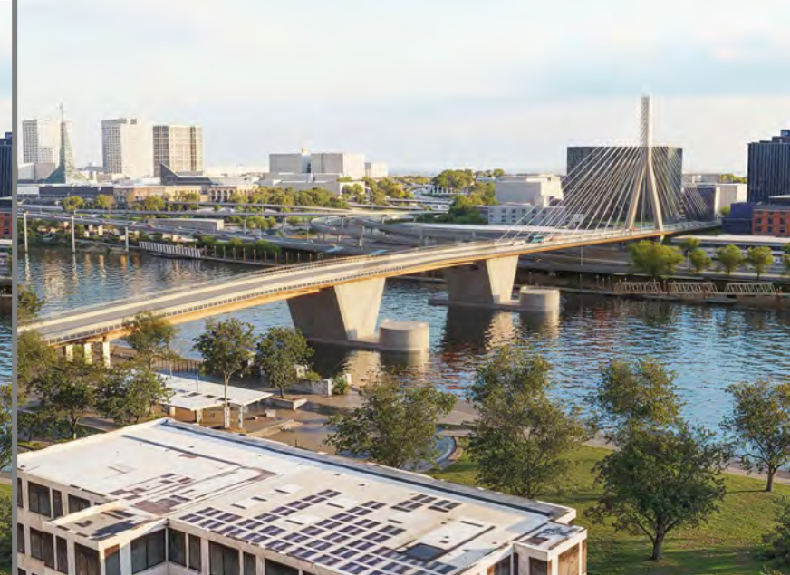
CS3- Inverted-Y tower
