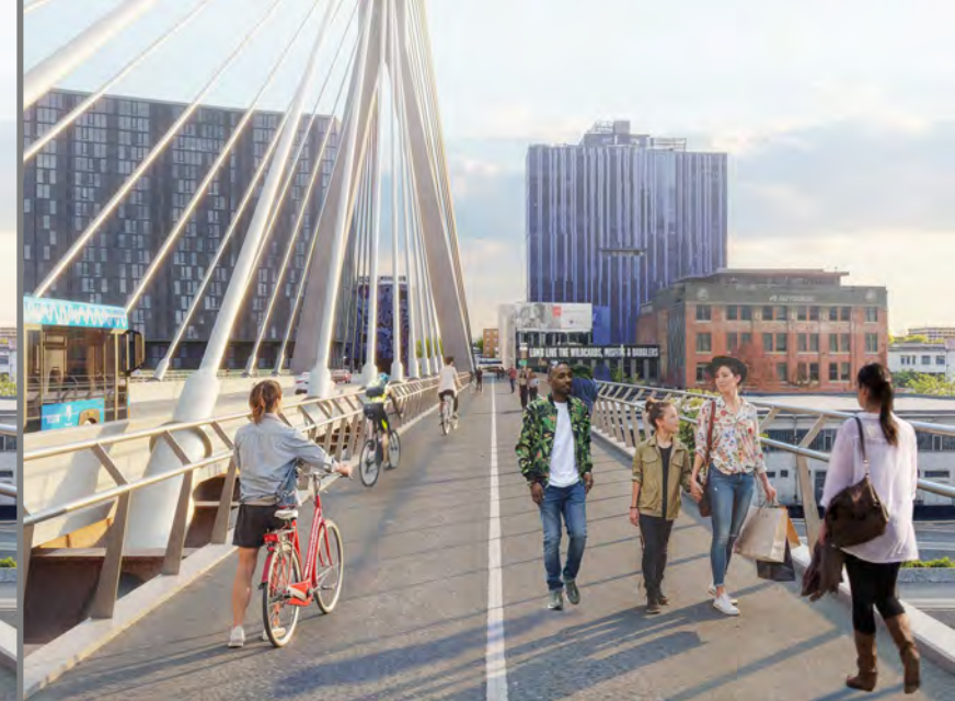
CS3- Inverted-Y tower
