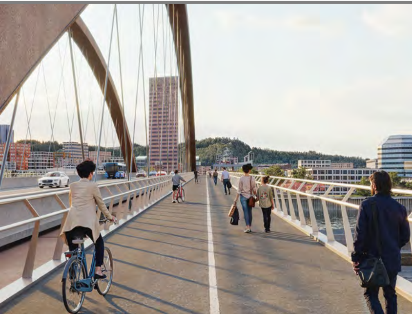
TA1-Unbraced vertical arches
