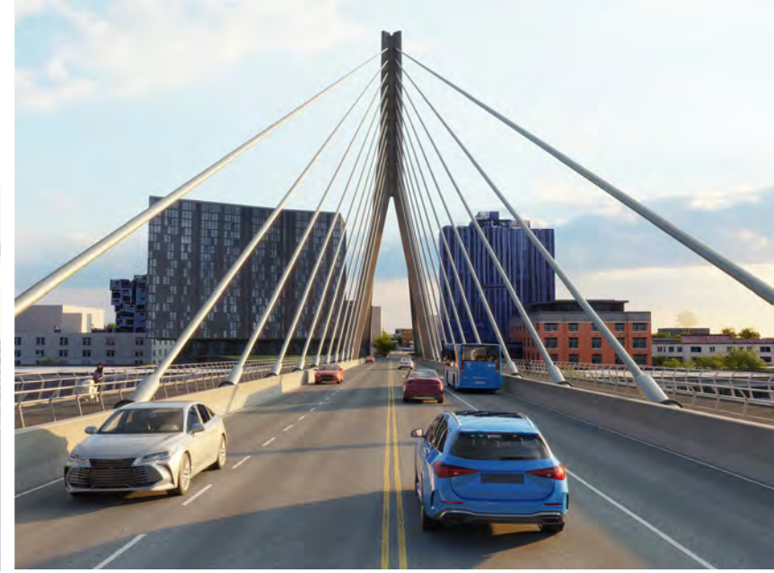
CS3- Inverted-Y tower
