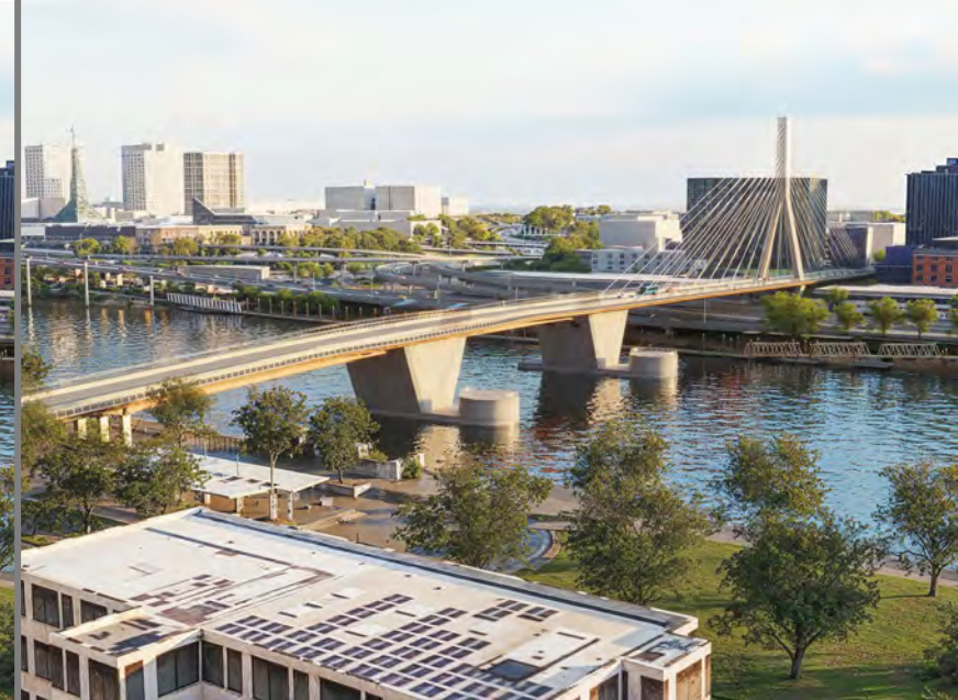
CS3- Inverted-Y tower
