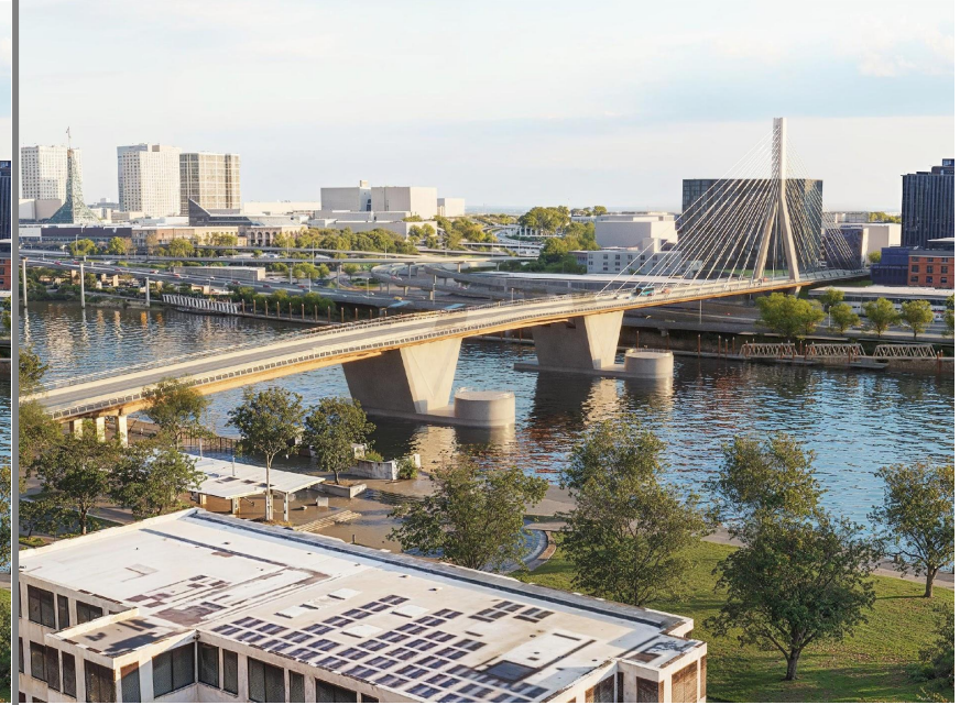
CS3- Inverted-Y tower
