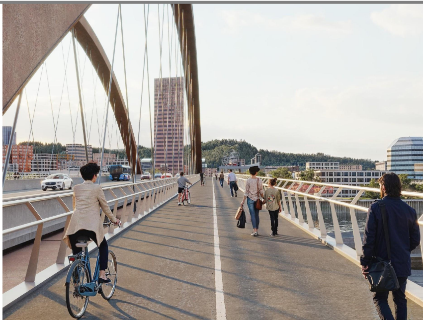
TA1-Unbraced vertical arches
