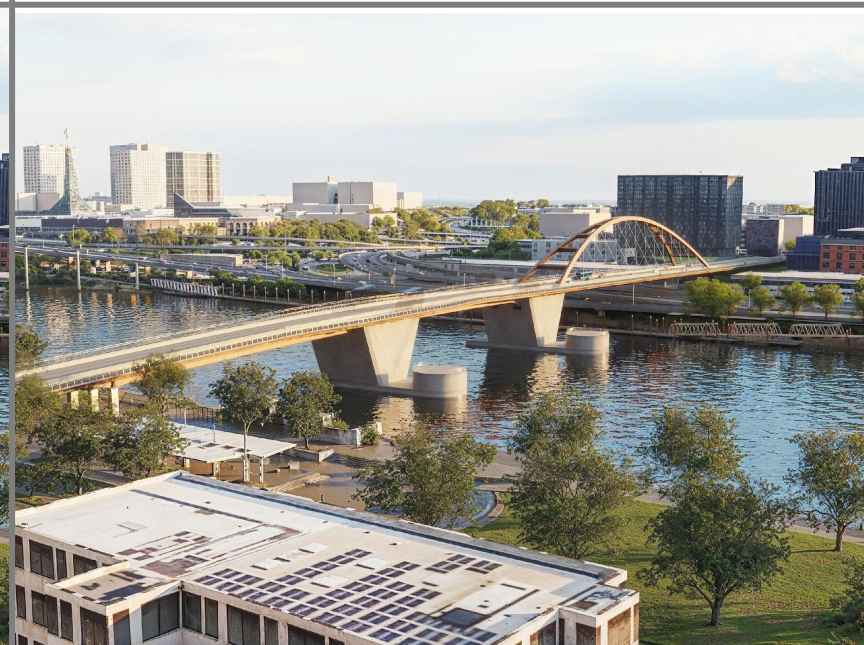
TA2-Braced basket-handle arch
