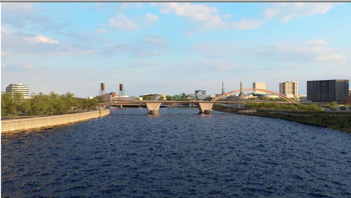
TA1-Unbraced vertical arches
