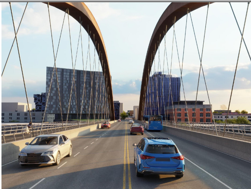
TA1-Unbraced vertical arches
