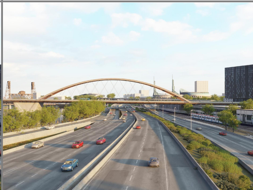
TA2-Braced basket-handle arch
