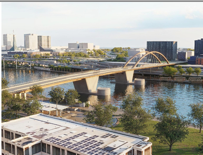
TA1-Unbraced vertical arches
