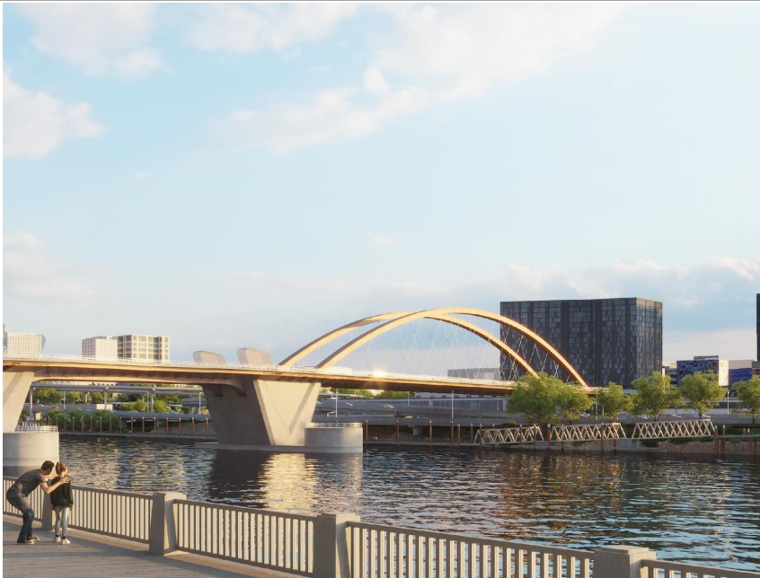
TA1-Unbraced vertical arches
