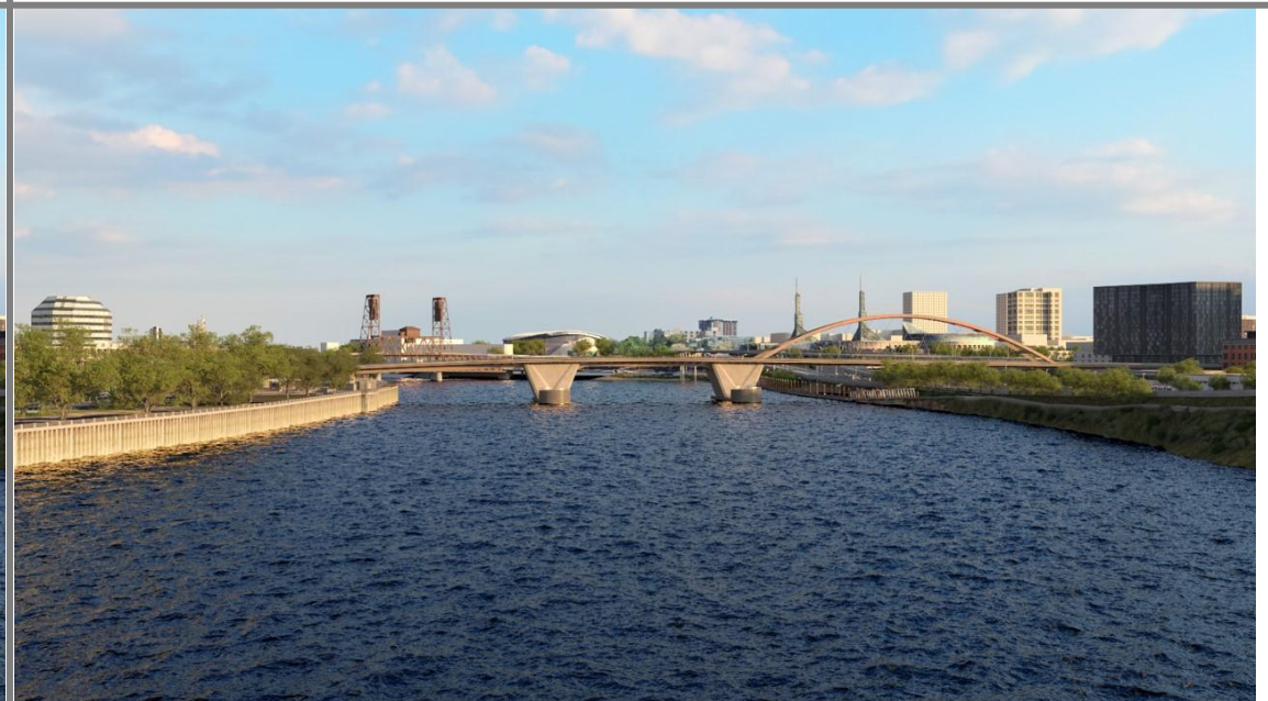
TA2-Braced basket-handle arch
