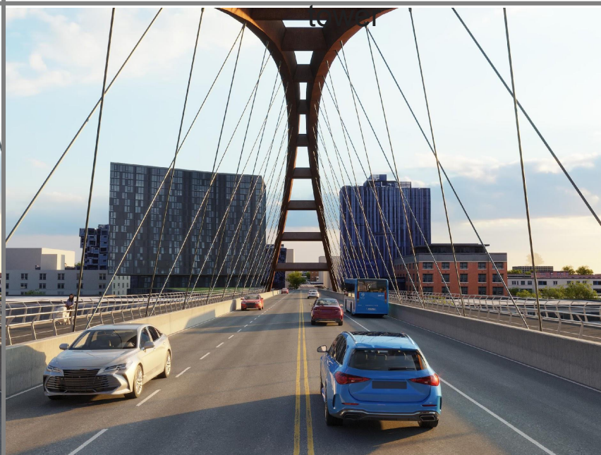
TA2-Braced basket-handle arch
