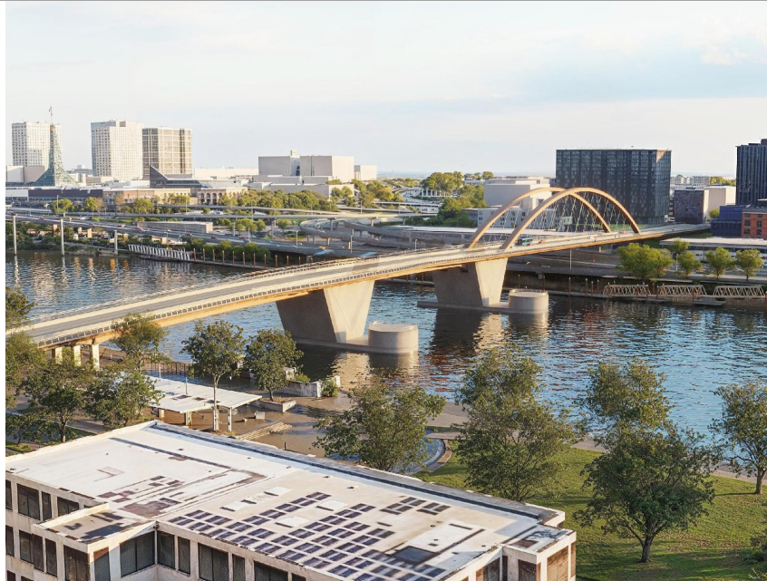
TA1-Unbraced vertical arches
