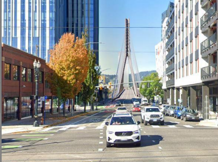
CS3- Inverted-Y tower
