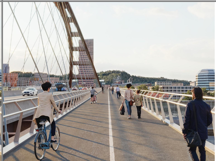
TA2-Braced basket-handle arch
