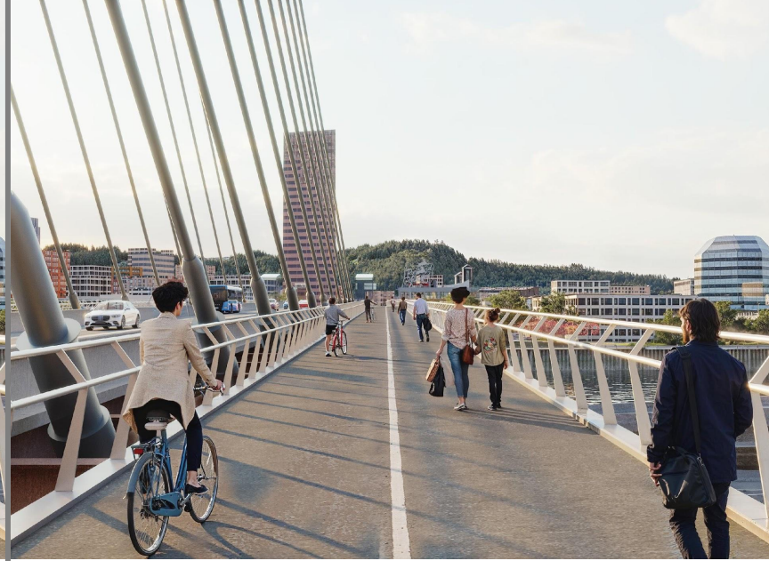
CS3- Inverted-Y tower
