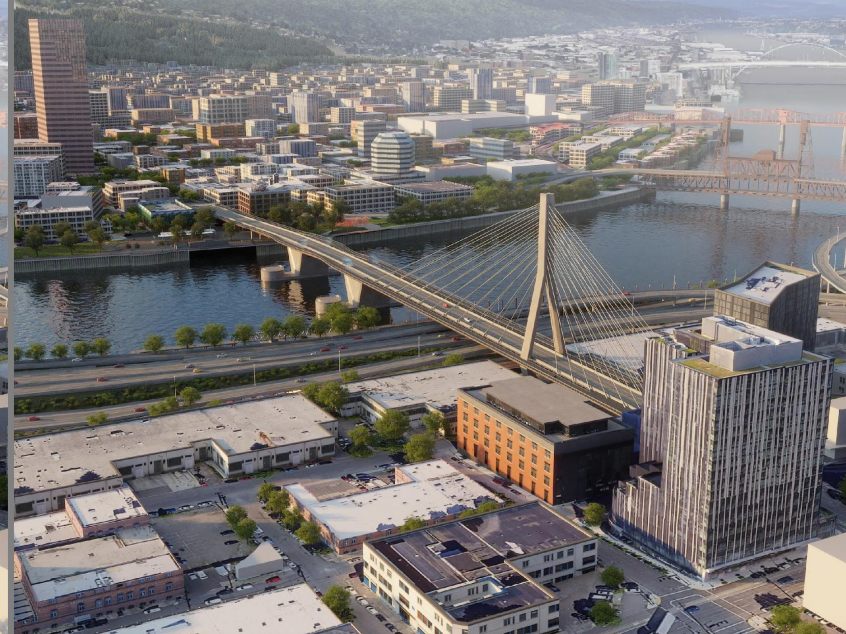
CS3- Inverted-Y tower
