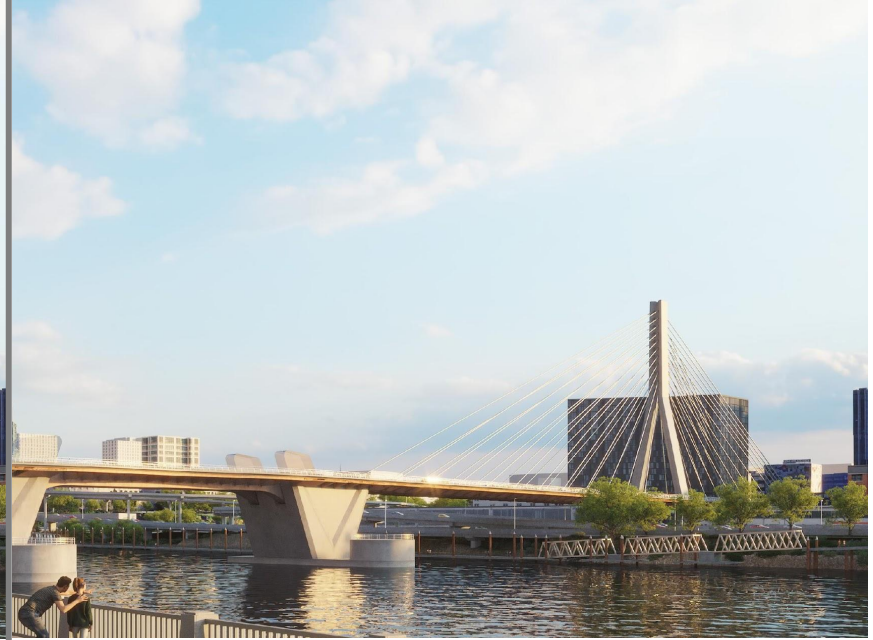
CS3- Inverted-Y tower
