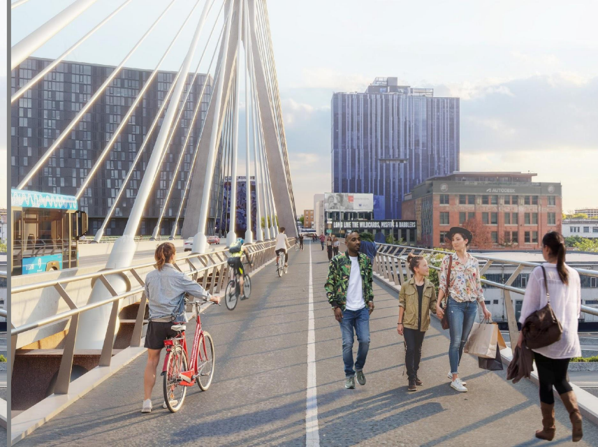
CS3- Inverted-Y tower
