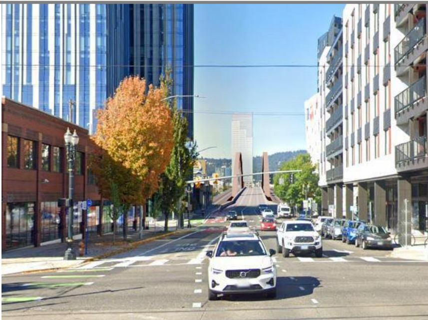
TA1-Unbraced vertical arches
