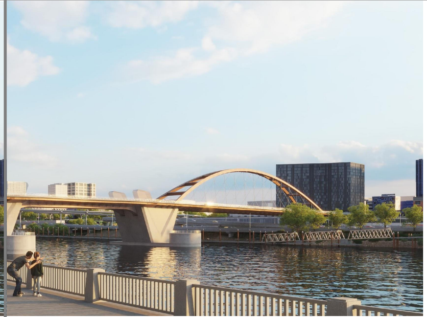
TA2-Braced basket-handle arch
