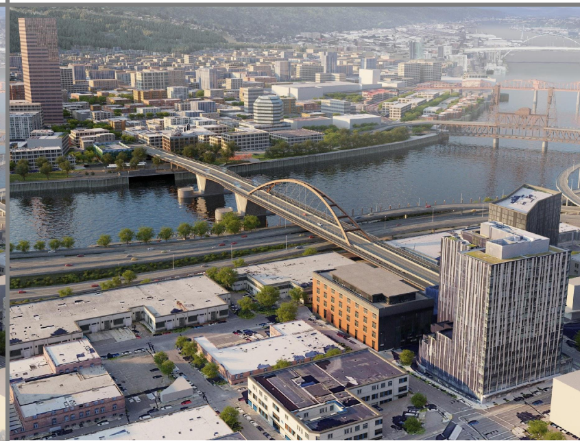
TA2-Braced basket-handle arch
