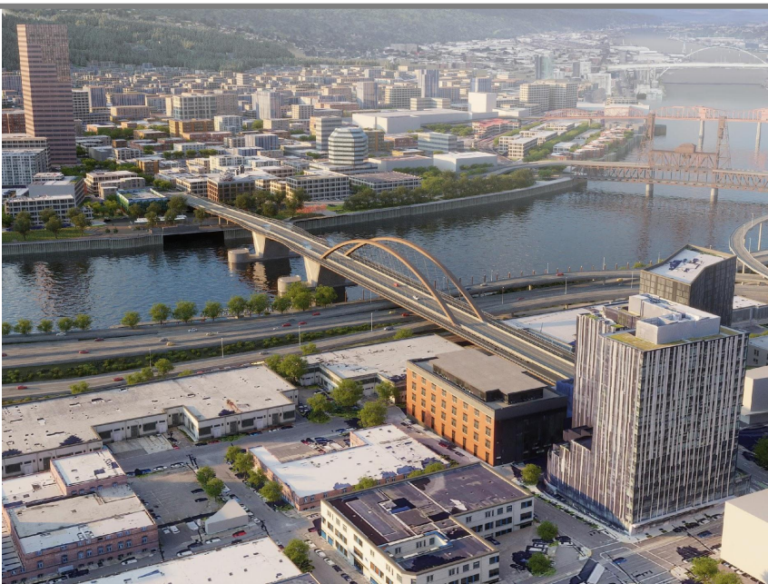
TA1-Unbraced vertical arches
