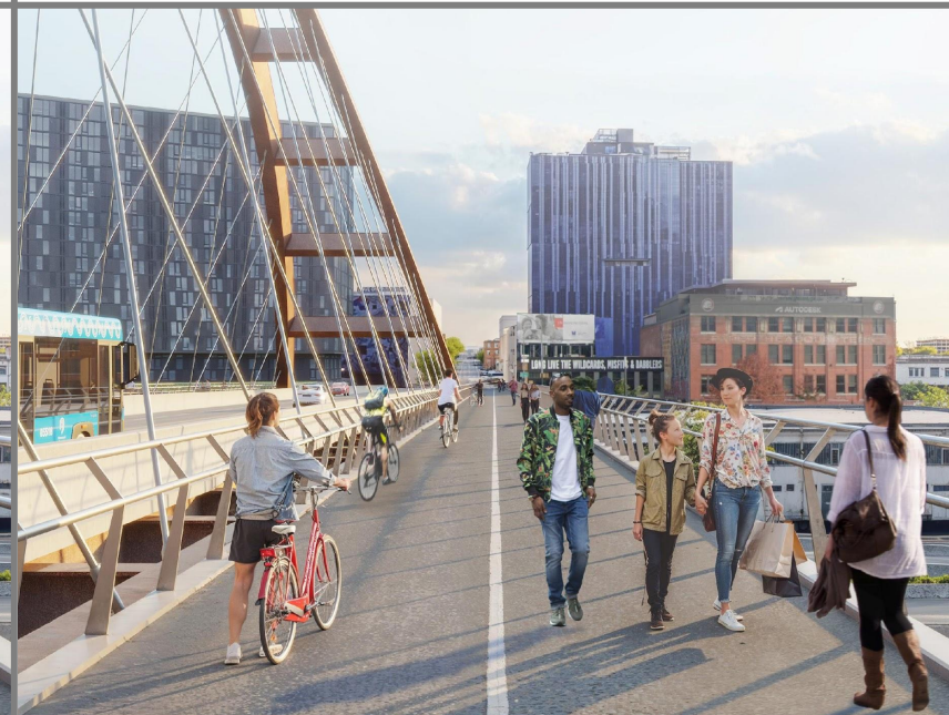
TA2-Braced basket-handle arch
