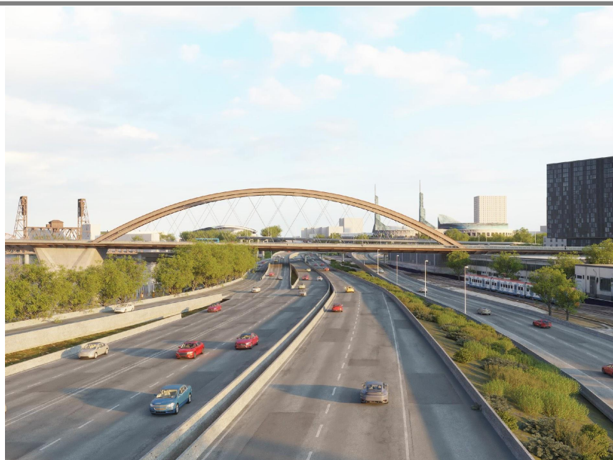
TA1-Unbraced vertical arches
