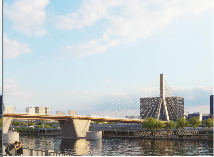
CS3- Inverted-Y tower
