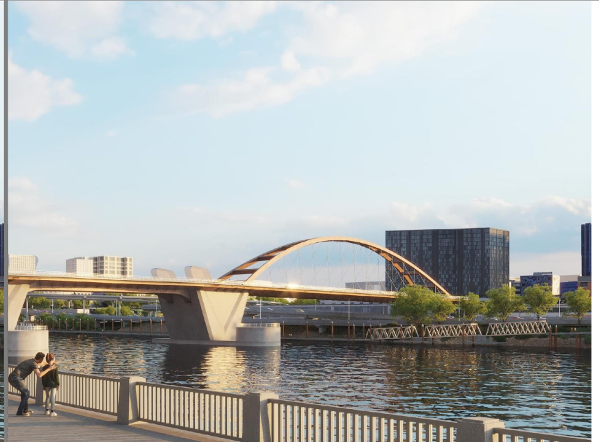
TA2-Braced basket-handle arch
