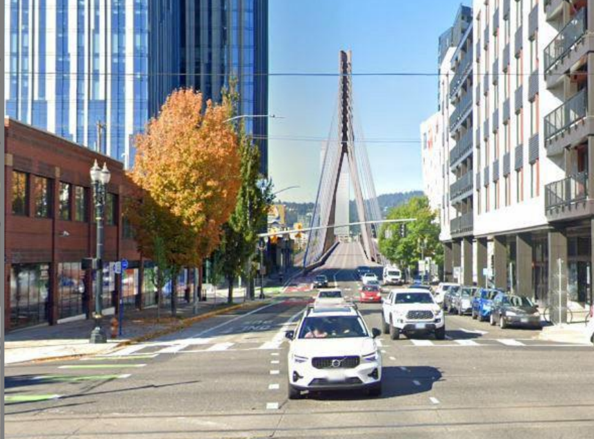
CS3- Inverted-Y tower
