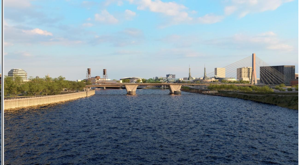
CS3- Inverted-Y tower
