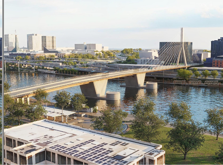
CS3- Inverted-Y tower
