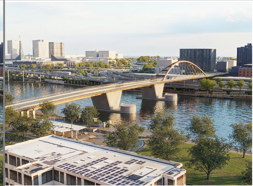
TA2-Braced basket-handle arch
