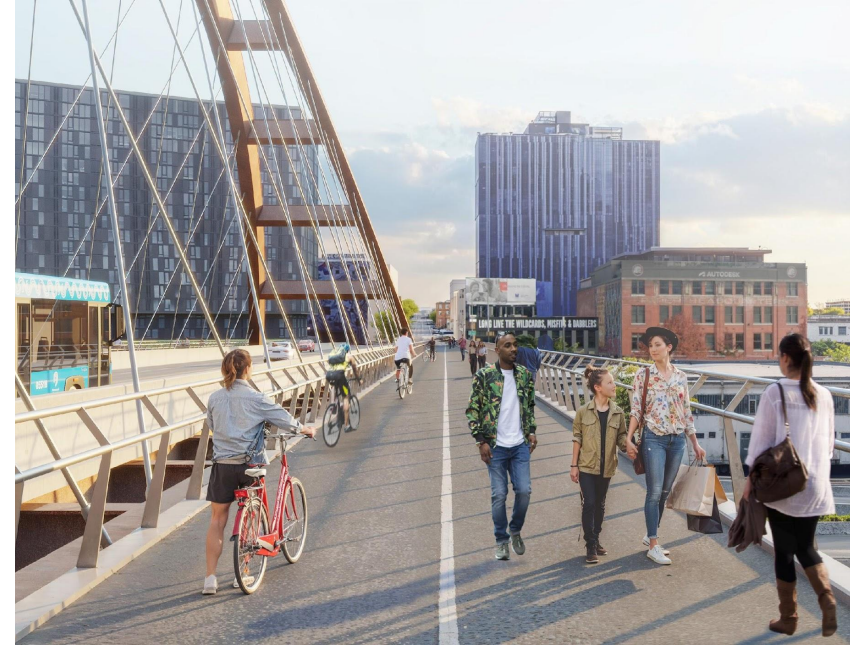
TA2-Braced basket-handle arch
