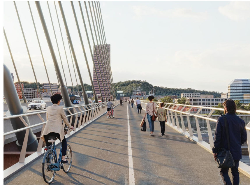
CS3- Inverted-Y tower
