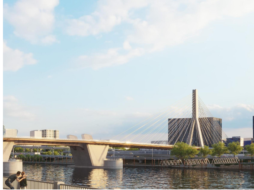
CS3- Inverted-Y tower
