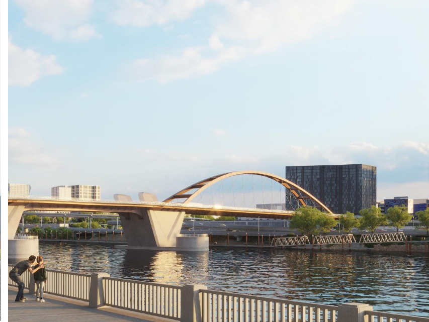
TA2-Braced basket-handle arch
