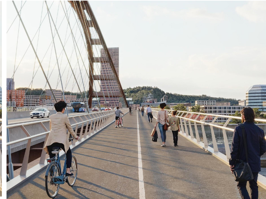
TA2-Braced basket-handle arch
