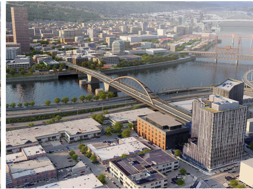
TA2-Braced basket-handle arch
