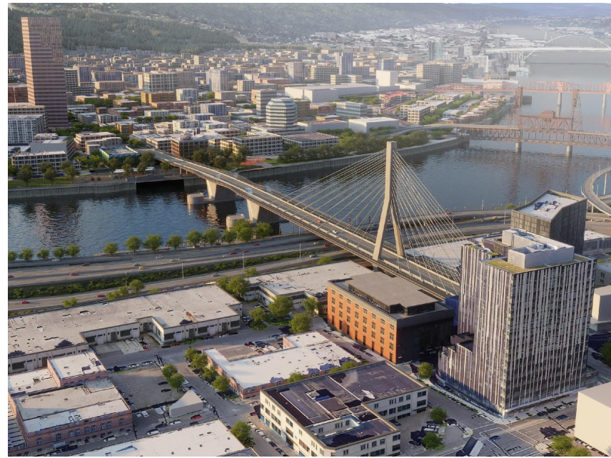
CS3- Inverted-Y tower
