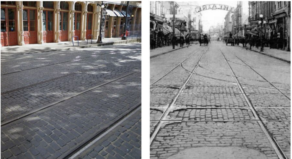
Cobblestone as paving surface:
