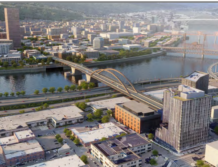
TA1-Unbraced vertical arches
