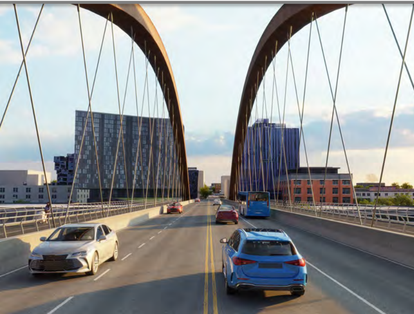
TA1-Unbraced vertical arches
