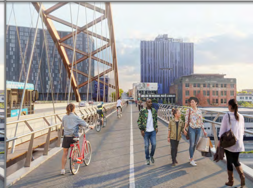
TA3- Braced vertical arches
