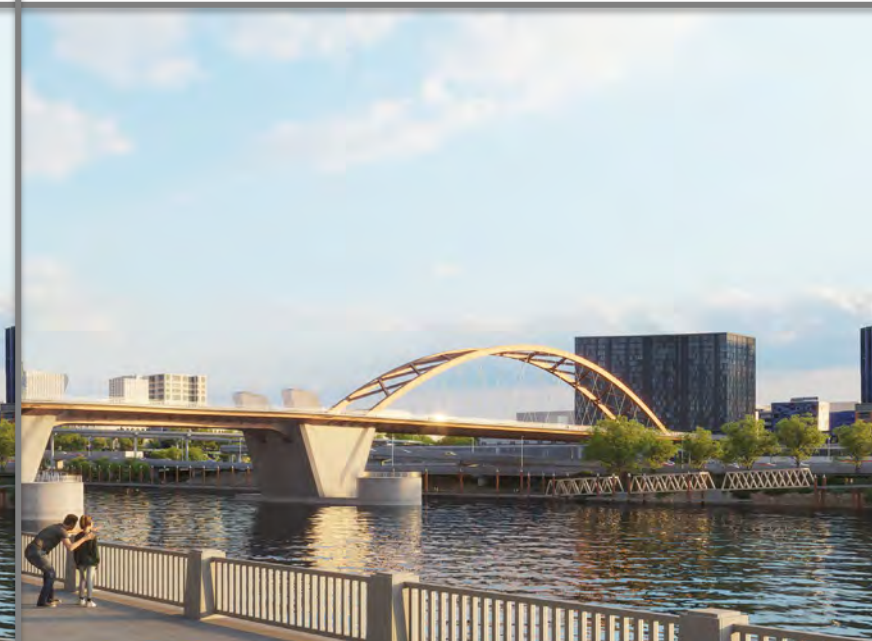
TA3- Braced vertical arches
