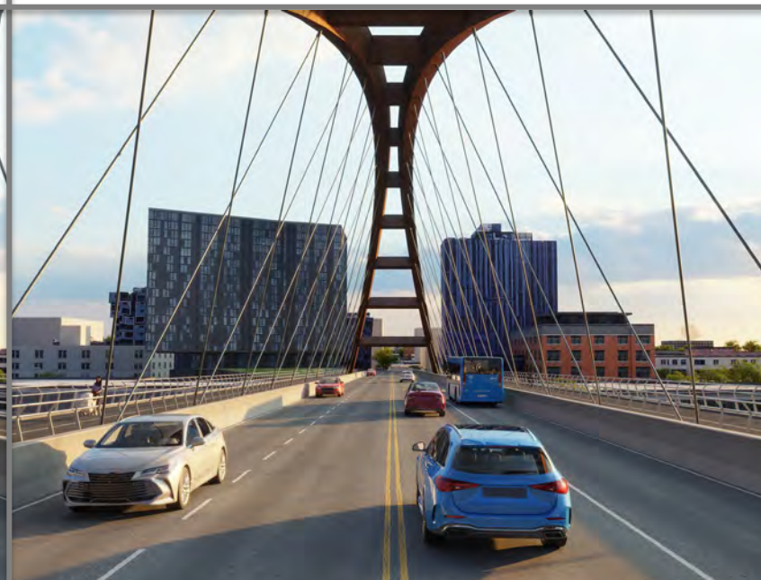
TA2-Braced basket-handle arch
