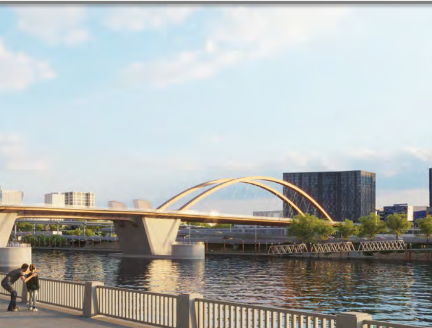
TA1-Unbraced vertical arches
