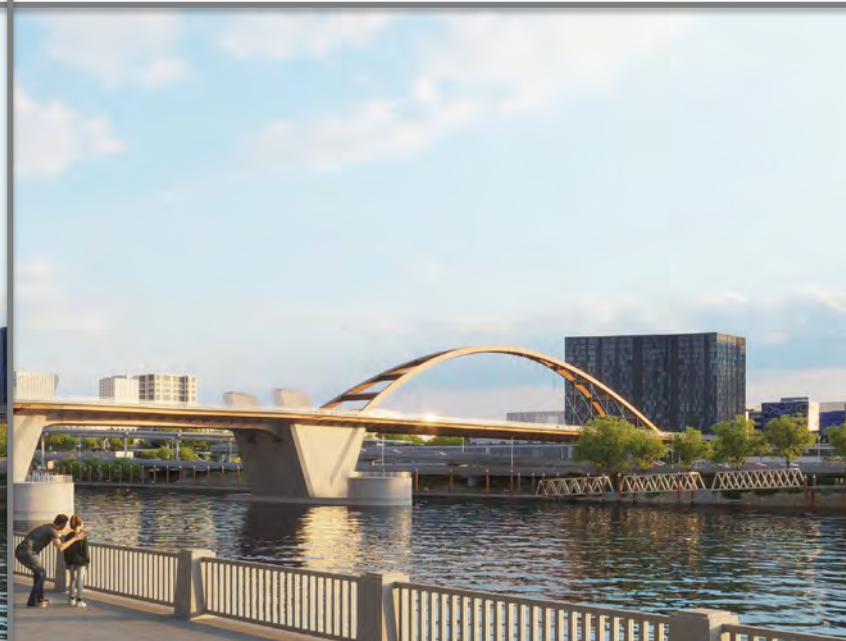
TA2-Braced basket-handle arch
