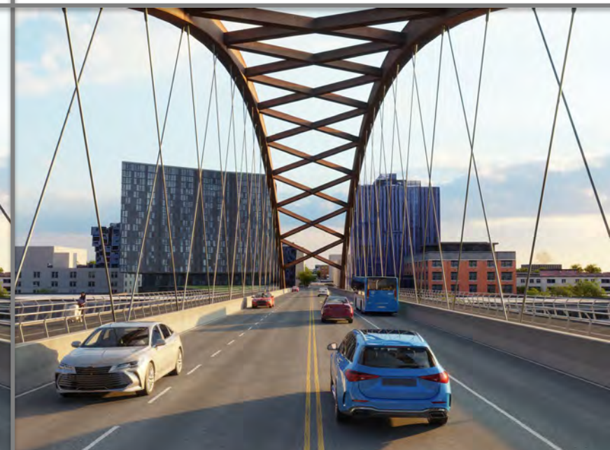
TA3- Braced vertical arches
