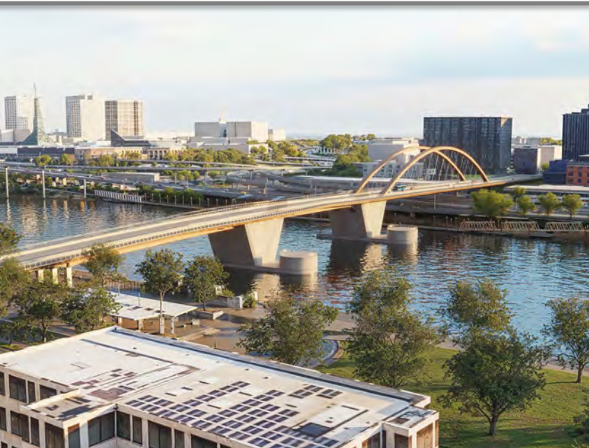
TA1-Unbraced vertical arches
