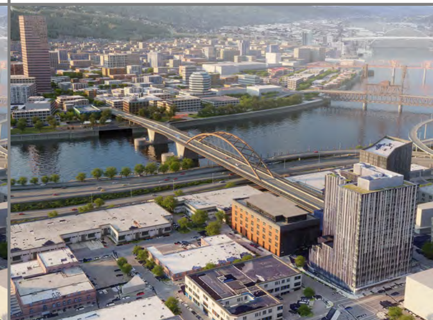
TA3- Braced vertical arches
