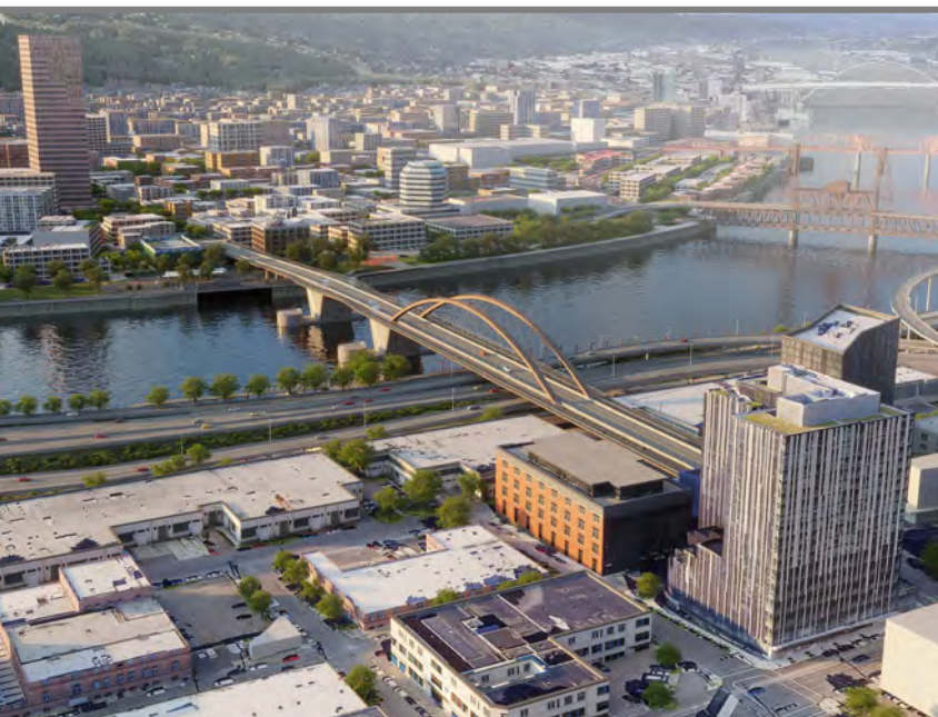
TA1-Unbraced vertical arches
