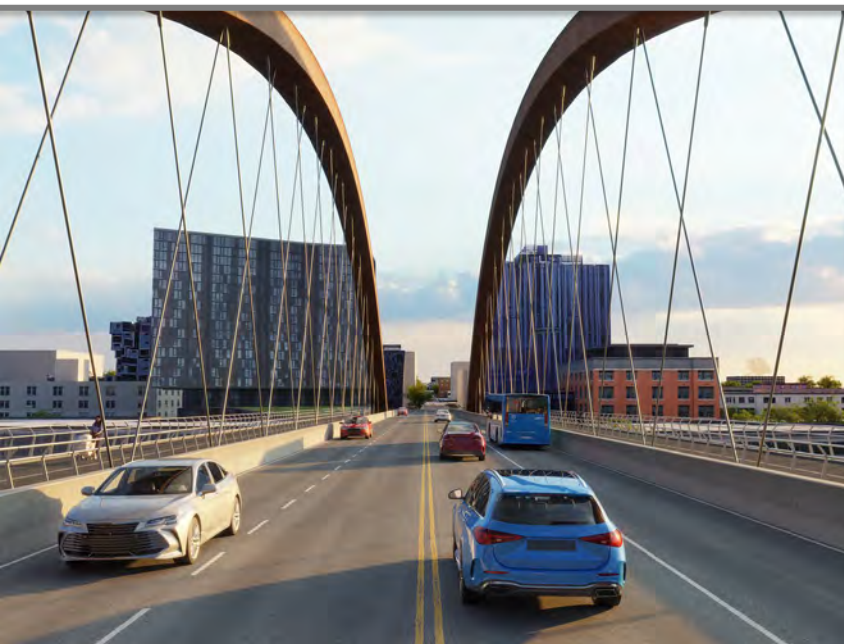
TA1-Unbraced vertical arches
