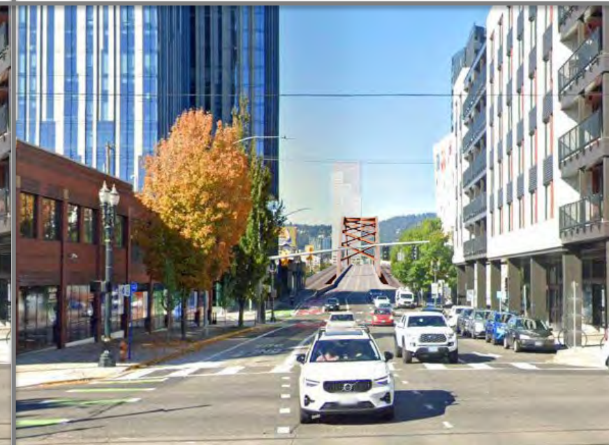
TA3- Braced vertical arches
