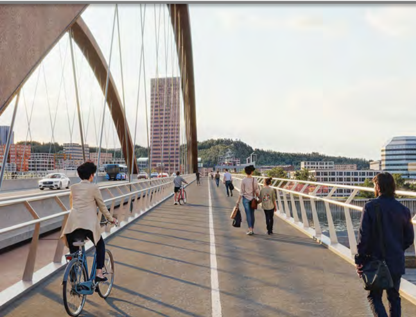
TA1-Unbraced vertical arches
