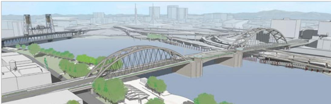
Figure 2.4-4. Refined Long-Span with Bascule Movable Span (Tied-Arch East Approach)
