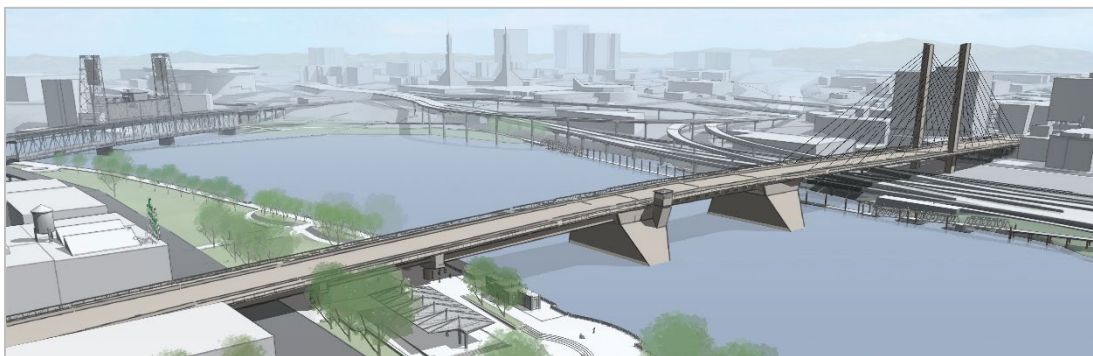
Figure 2.4-6. Refined Long-Span Cable with Bascule Lift Movable Span (Cable-Stayed East Approach)
