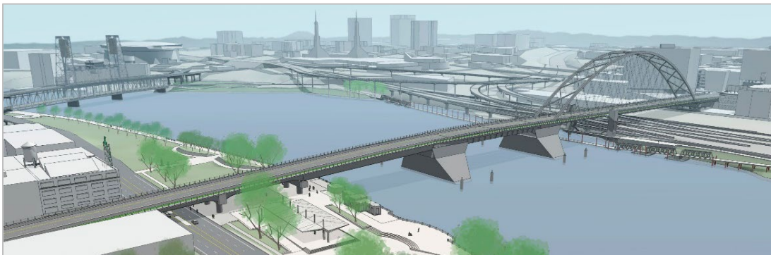
Figure 2.4-4. Refined Long-Span with Bascule Movable Span (Tied-Arch East Approach)
