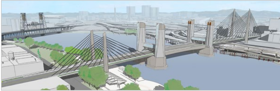
Figure 2.4-6. Refined Long-Span Cable with Bascule Lift Movable Span (Cable-Stayed East Approach)
